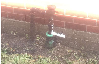
Vacuum Breaker/Backflow Preventer: Installed
