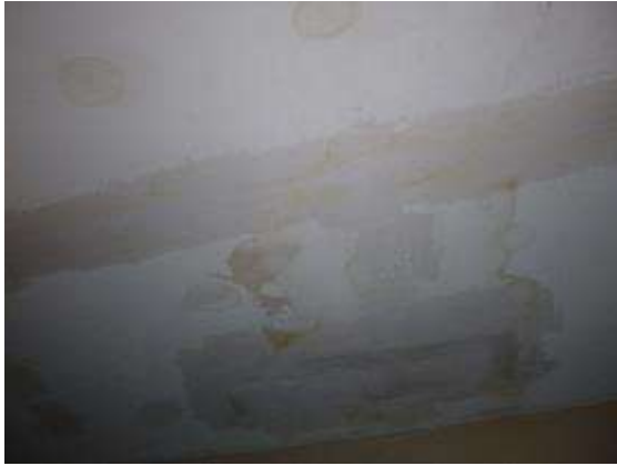
Unit A kitchen ceiling
