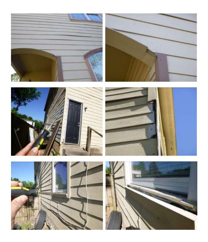
The siding around the house was loose/warped and need to be resecured. **Obtain Cost Estimate**
