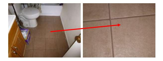
Floor tiles were loose and need to be repaired. **Obtain Cost Estimate**
