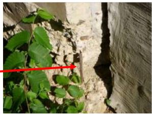
We observed wood form boards at the face of the foundation and it is recommended that the form boards be removed to eliminate a conducive condition for infestation by wood destroying insects.
