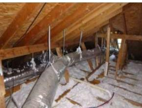
Wind uplift or hurricane clips and/or straps were observed to be installed over the ridge beam to rafters on both sides of the ridge beam, and also at the hip rafters. This provides a stronger structure and will be more resistant to wind uplift from hurricane and tornadoes. Due to the insulation installed at the eaves of the attic, we were not able to view the metal clips attaching the rafters to the top of the wall framing.
