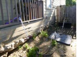
The face of the foundation concrete was spalled, and the reinforcing steel used in the construction of the foundation was observed to be exposed. The rust should be removed from the rebar, and the rebar grouted to prevent further deterioration.
