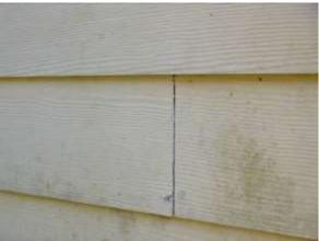
The siding around the house was damaged/broken and needs to be repaired.
