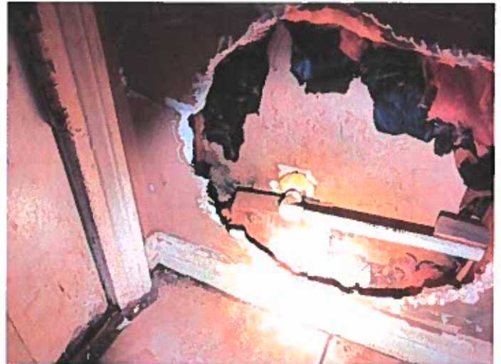
Laundry room wall
