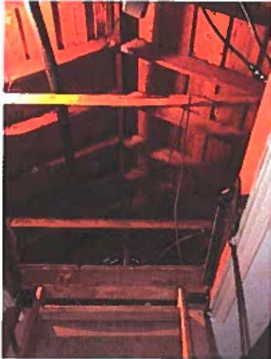
Rafters without adequate collar ties
