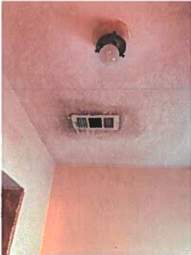
Hall bathroom ceiling
