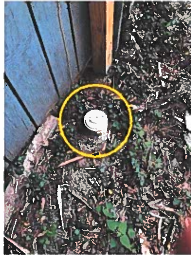
Waste cleanout located at rear of garage
