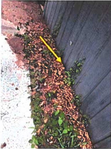
Siding at garage
