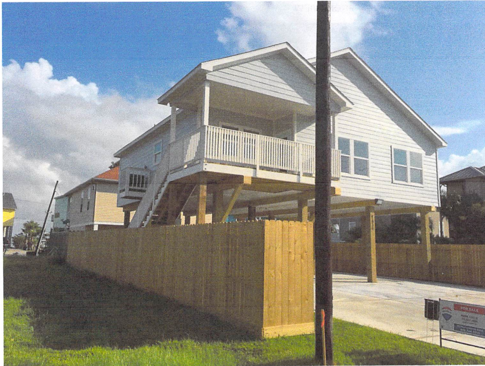
Picture Taken: Jul 31, 2019 WEST SIDE VIEW
