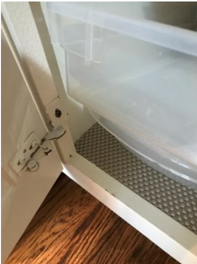
Loose door hinge noted on the base cabinet Ashanti the refrigerator.
