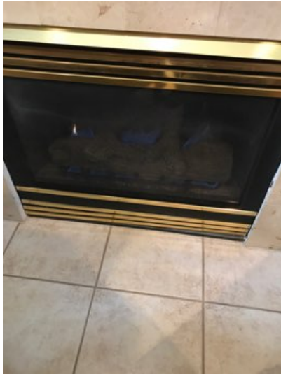
Structural Systems Fireplace/Chimney
