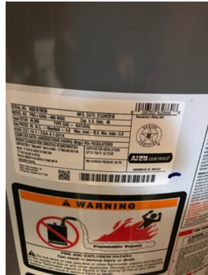
Plumbing Systems Water Heating Equipment
