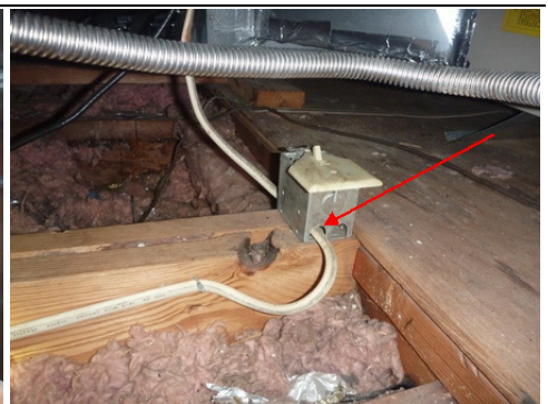
*Install insulator at knockout
