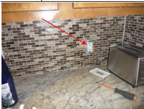
*Install box extenders
