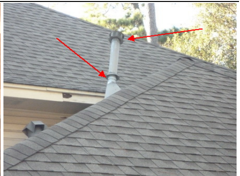
*Adjust storm collar and breather cap
