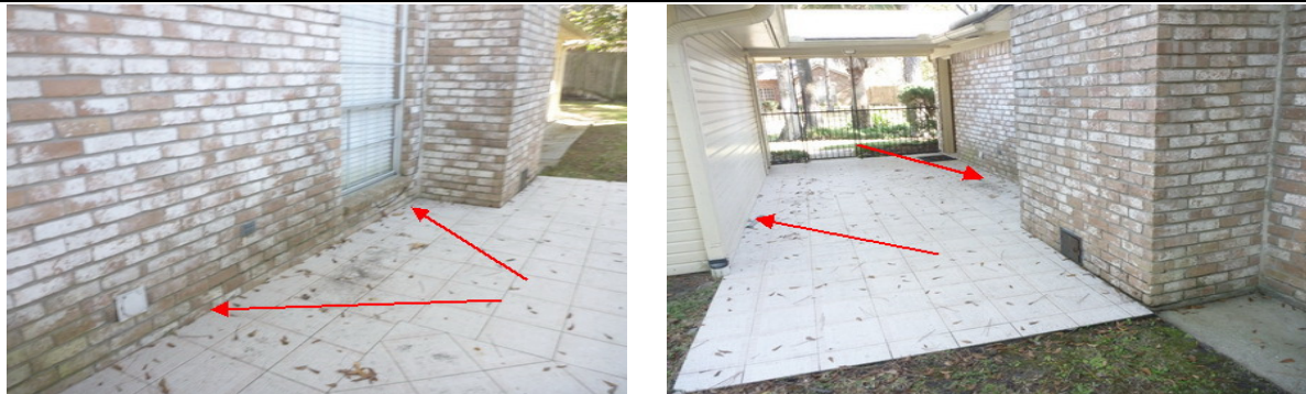
*Patio flooring installed over the exterior finish wall materials
