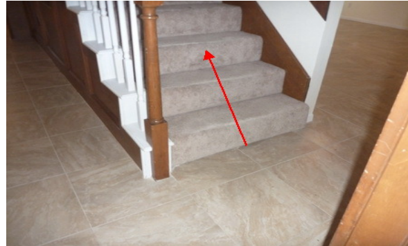
*The baluster spacing exceeds 4"; the handrails should return back to the side walls; riser height variance
