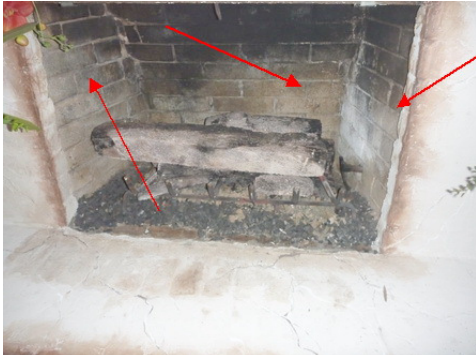
*Evidence of water /moisture seepage into the firebox. *Install metal cap flashings at the horizontal masonry surfaces
