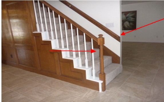
*The baluster spacing exceeds 4"; the handrails should return back to the side walls; riser height variance
