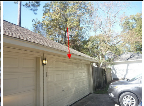
*Moisture damaged base trim-left rear 1 st floor **Redo brick veneer *OH garage door frame header deflection
