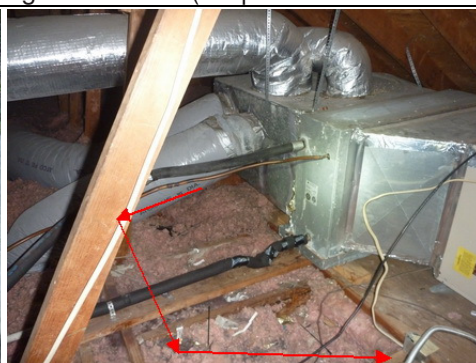
*Provide a walk path/ work platform
