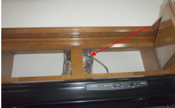
*Seal vent pipe in cabinet and solid smooth wall piping is required thru to the exterior
