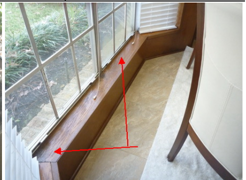
*Evidence of water leaking-top of windows *Interior sills/ possible frame damage – front room and breakfast area
