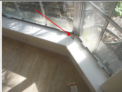
*Evidence of water leaking-top of windows *Interior sills/ possible frame damage – front room and breakfast area
