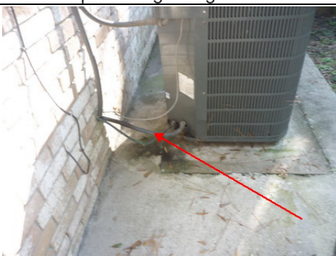
*Insulate the refrigerant line
