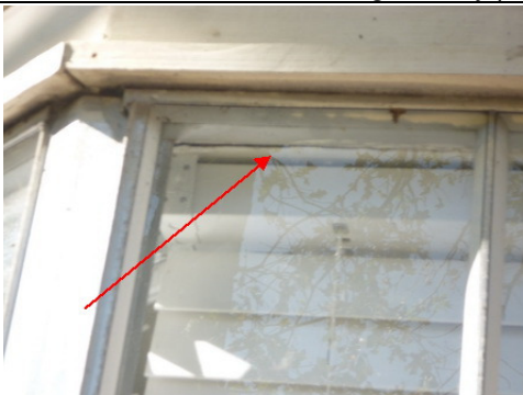
*Evidence of water leaking-top of windows *Interior sills/ possible frame damage – front room and breakfast area
