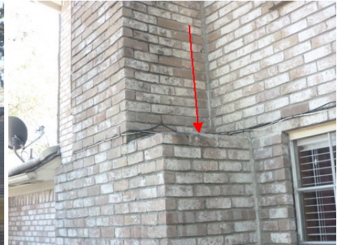
*Evidence of water /moisture seepage into the firebox. *Install metal cap flashings at the horizontal masonry surfaces
