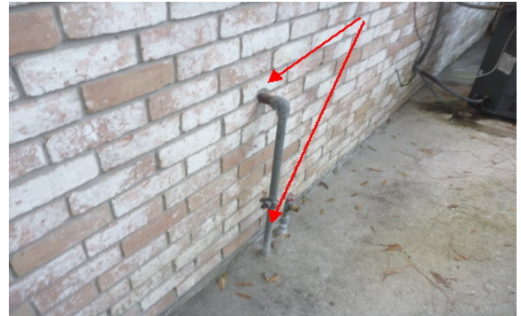
*Install protective sleeves for the gas pipe
