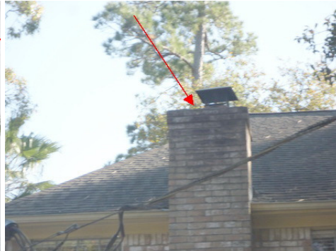
*Evidence of water /moisture seepage into the firebox. *Install metal cap flashings at the horizontal masonry surfaces
