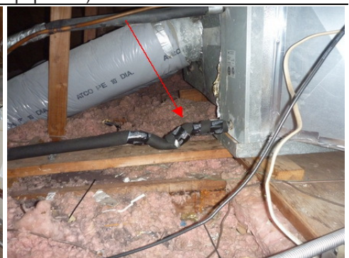
*Install a riser vent
