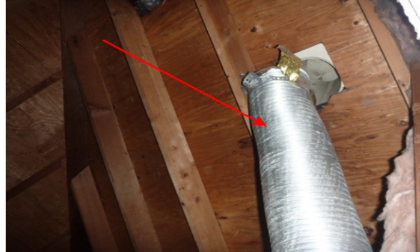
*Seal vent pipe in cabinet and solid smooth wall piping is required thru to the exterior
