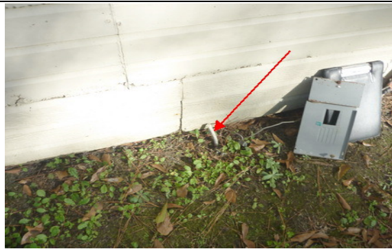
*Rust / water entry into panel; missing insulator; drive ground rod fully into earth
