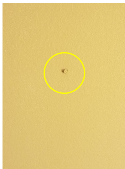
Exposed or protruding drywall fasteners were noted on the 2nd level.
