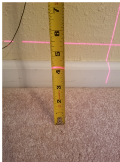
Some floor differential was noted in the 2nd level den. It is not uncommon for 2nd levels to show some differential, however, these measurements could be significant. For further evaluation we recommend consulting with a qualified contractor.
