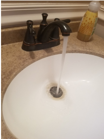
Sink stopper not working/missing in the 2nd level half bathroom and master bathroom. Flex drain piping was observed at some traps and is easily clogged.
