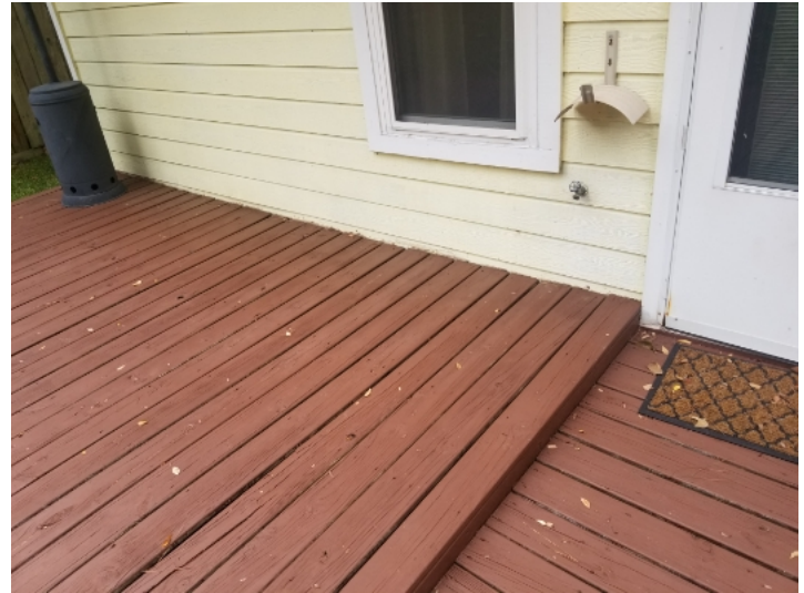
Some of the foundation was not visible due to decking.
