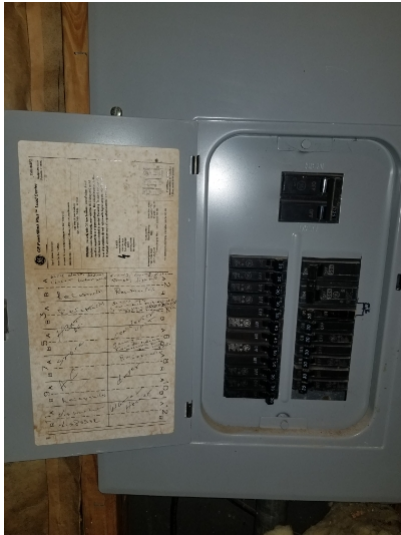
Electrical Systems Service Entrance and Panels All breakers for the panel boxes and/or sub panels must be clearly and permanently labeled for identification of particular circuit.
