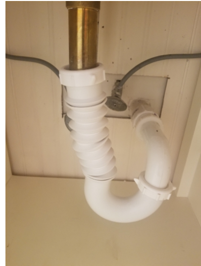
Sink stopper not working/missing in the 2nd level half bathroom and master bathroom. Flex drain piping was observed at some traps and is easily clogged.
