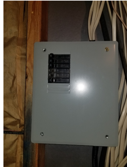
Electrical Systems Service Entrance and Panels All breakers for the panel boxes and/or sub panels must be clearly and permanently labeled for identification of particular circuit.
