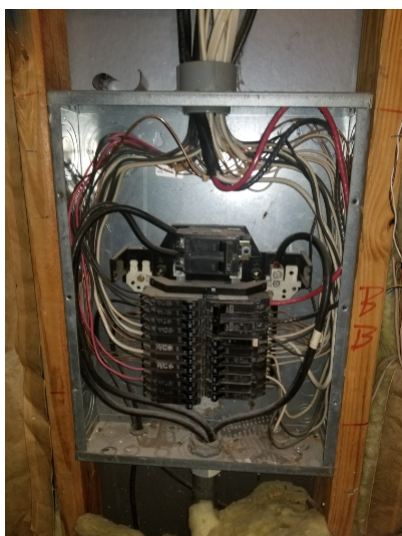
Electrical Systems Service Entrance and Panels White wires were connected directly to breakers in the panel. Typically white wires should be designated as neutral only. These should be marked appropriately.
