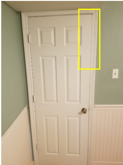
The 1st level bathroom and front bedroom doors were not square and contacting the frame and may require adjustment.
