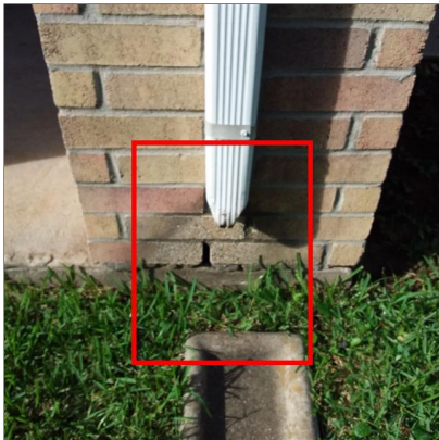
B. Item 2(Picture) Front left side of home
