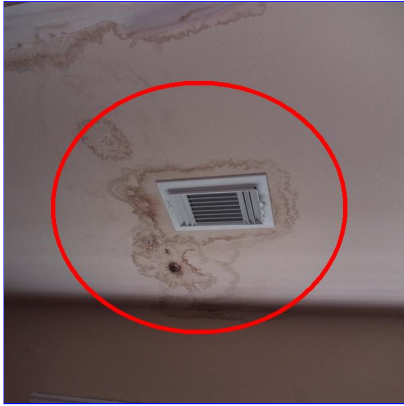
F. Item 32(Picture) Right side of downstairs bedroom
