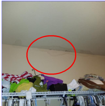
E. Item 43(Picture) Right side of master bedroom closet
