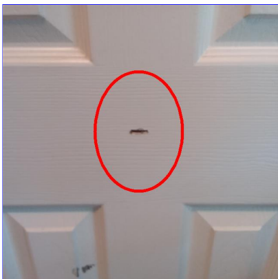
G. Item 6(Picture) Main entry closet
