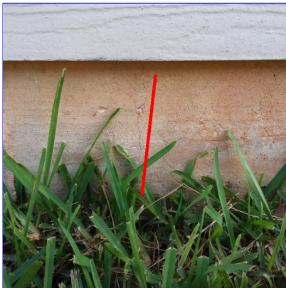
A. Item 3(Picture) Right side of home
