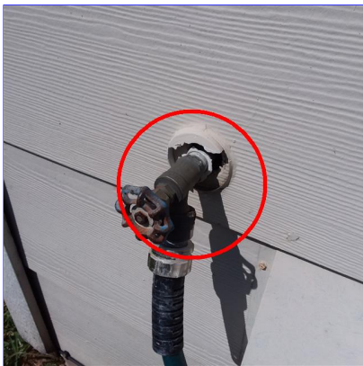
E. Item 7(Picture) Right rear of home
