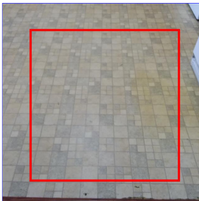
F. Item 2(Picture) Kitchen
