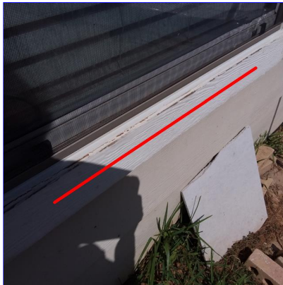
E. Item 2(Picture) Right rear of home
