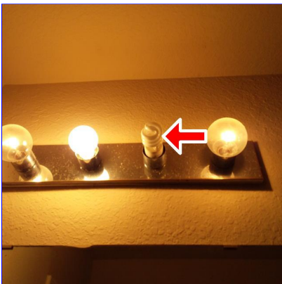
B. Item 5(Picture) Hall bath
