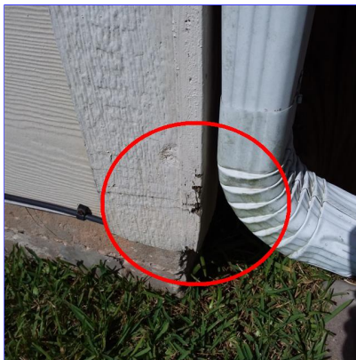
E. Item 19(Picture) Left rear of home
