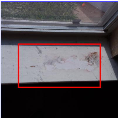
H. Item 11(Picture) Right rear of living room
