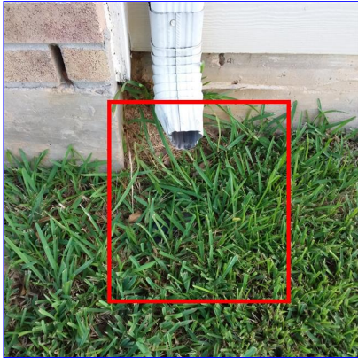
B. Item 1(Picture) Front right side of home
