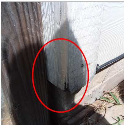
E. Item 18(Picture) Right rear of home
