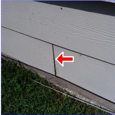
E. Item 50(Picture) Left rear of home
