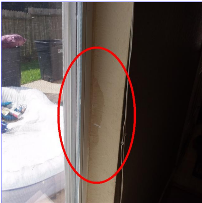
H. Item 9(Picture) Right rear of living room
