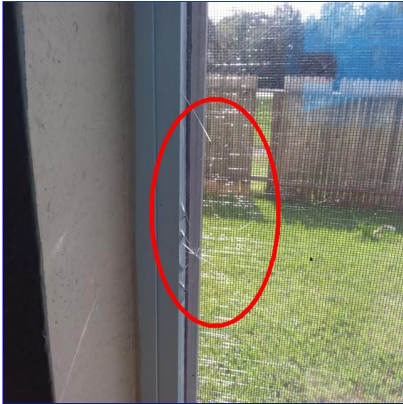
H. Item 8(Picture) Right rear of living room
