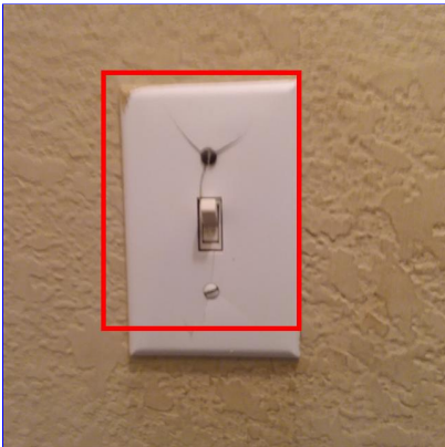
B. Item 7(Picture) Garage entry
