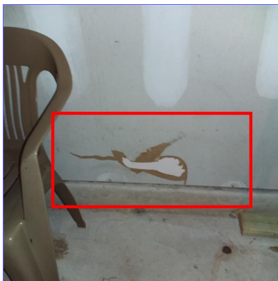
E. Item 27(Picture) Left side of garage
