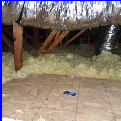
Blown insulation
