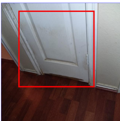
G. Item 8(Picture) Upstairs front hall closet
