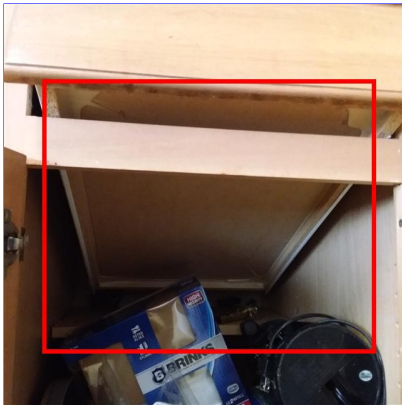
I. Item 5(Picture) Front right side of kitchen
