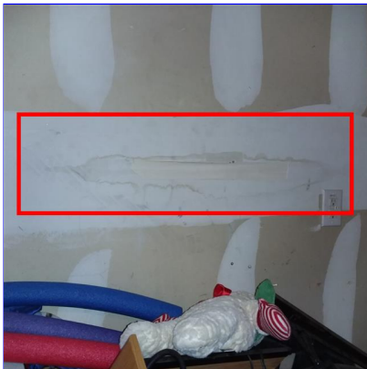
E. Item 39(Picture) Rear of garage
