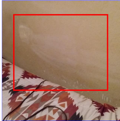
E. Item 29(Picture) Rear of left rear bedroom
