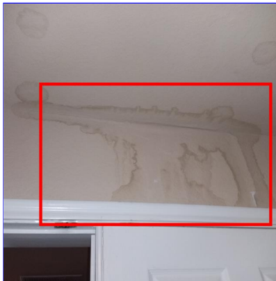
E. Item 40(Picture) Left side of downstairs bedroom
