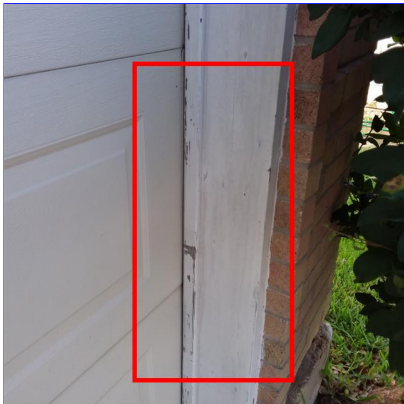
E. Item 1(Picture) Front right of home
