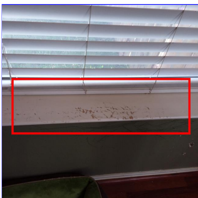
H. Item 7(Picture) Left rear side of living room
