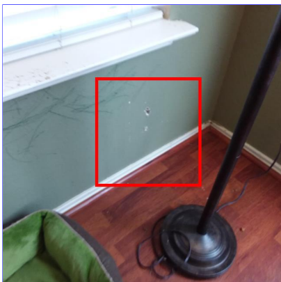
E. Item 26(Picture) Left rear side of living room
