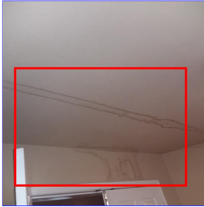
F. Item 33(Picture) Left side of downstairs bedroom
