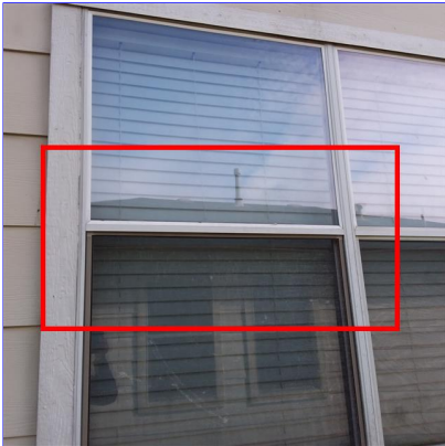
H. Item 1(Picture) Right side of home
