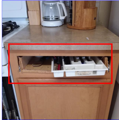
I. Item 4(Picture) Front of kitchen
