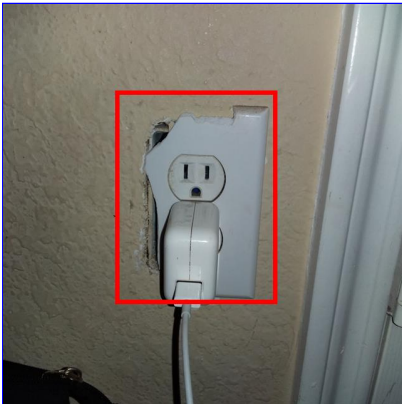
B. Item 16(Picture) Right side of front left bedroom
