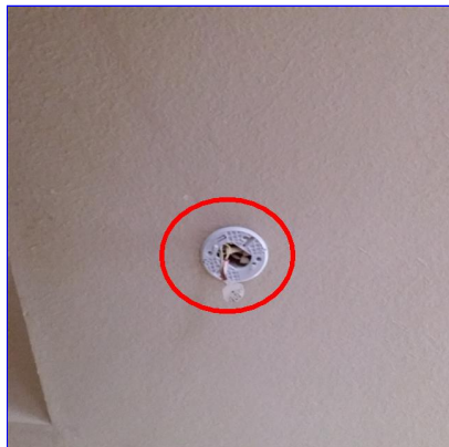
B. Item 10(Picture) Lower level stairway entry
