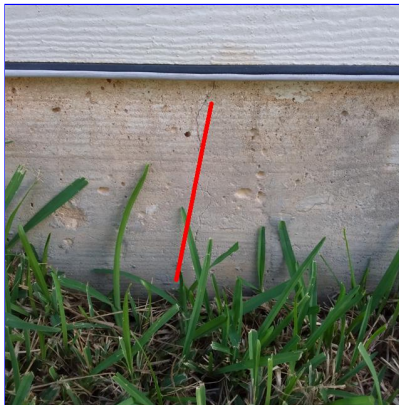
A. Item 4(Picture) Right side of home
