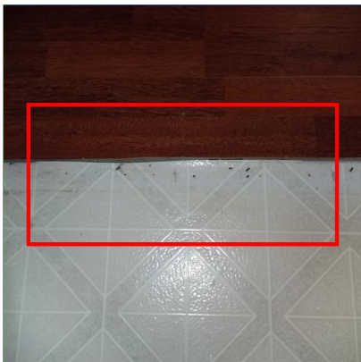
F. Item 18(Picture) Washer/dryer room entry
