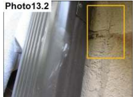
Control Joint Cracks/ Seal
