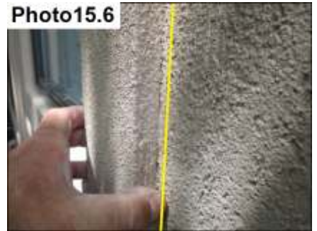
Window Trim/Stucco Termination Sealants/ Seal
