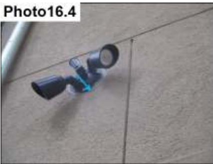
Penetration Sealants/ Maintain
