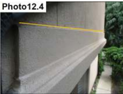
Foam/Stucco Termination Sealants/ Seal
