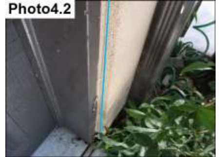
Door Trim Sealants/ Maintain
