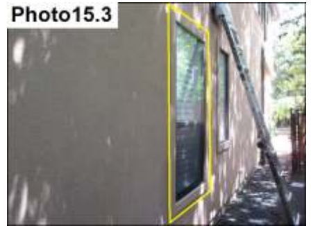
Window Trim/Stucco Termination Sealants/ Seal
