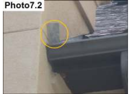
Kickout Flashing Sealants/ Seal
