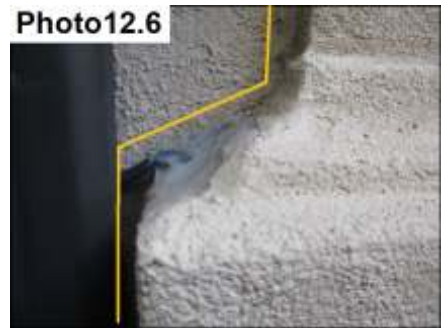
Foam/Stucco Termination Sealants/ Seal
