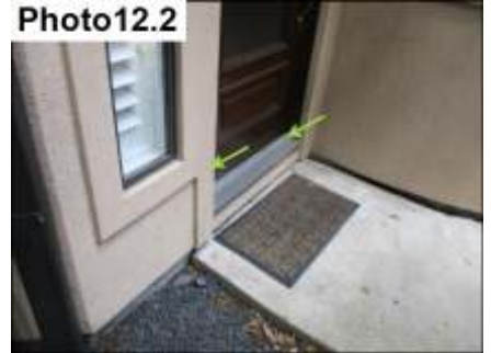
Door Trim And Miter Sealants/ Maintain
