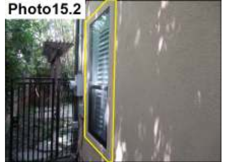
Window Trim/Stucco Termination Sealants/ Seal
