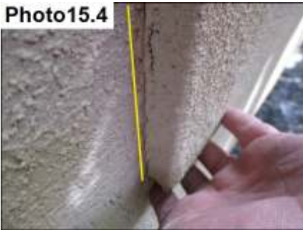
Window Trim/Stucco Termination Sealants/ Seal
