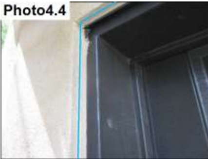
Door Trim Sealants/ Maintain
