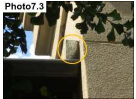
Kickout Flashing Sealants/ Seal
