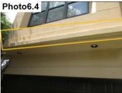
Photo6.4 Semi-Firm Substrate/ Install Relief
