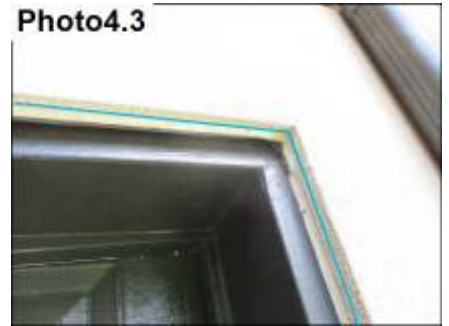
Door Trim Sealants/ Maintain
