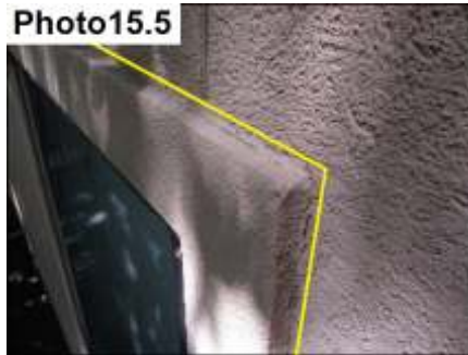
Window Trim/Stucco Termination Sealants/ Seal
