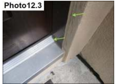
Door Trim And Miter Sealants/ Maintain
