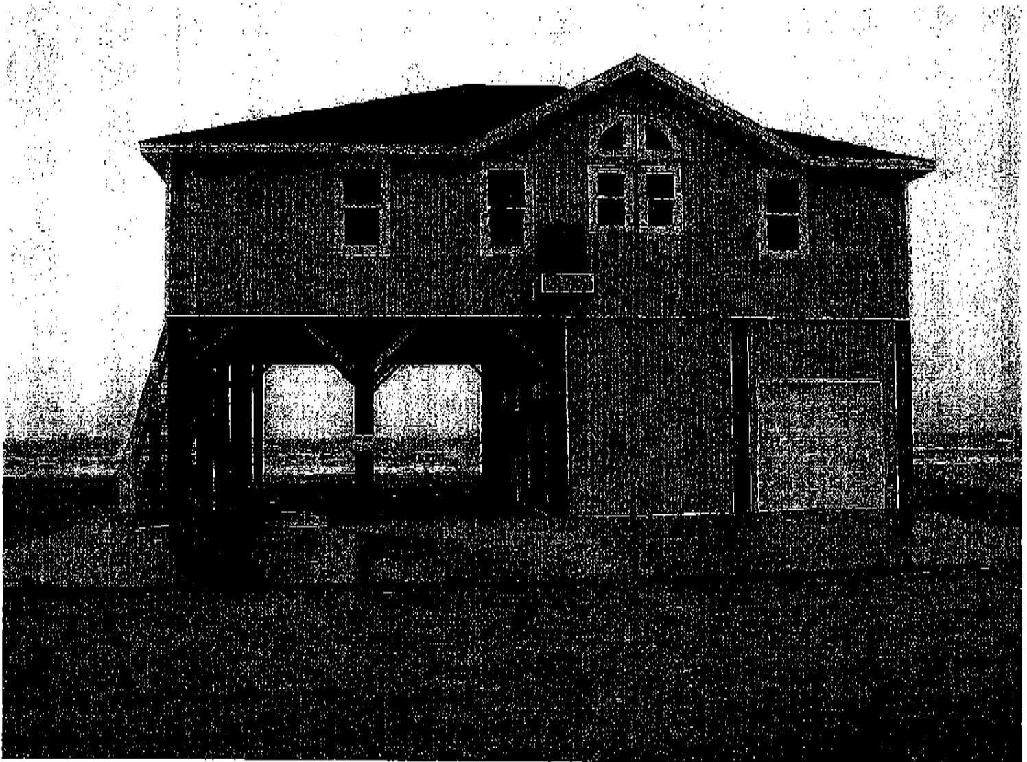
FRONT VIEW OF BUILDING
