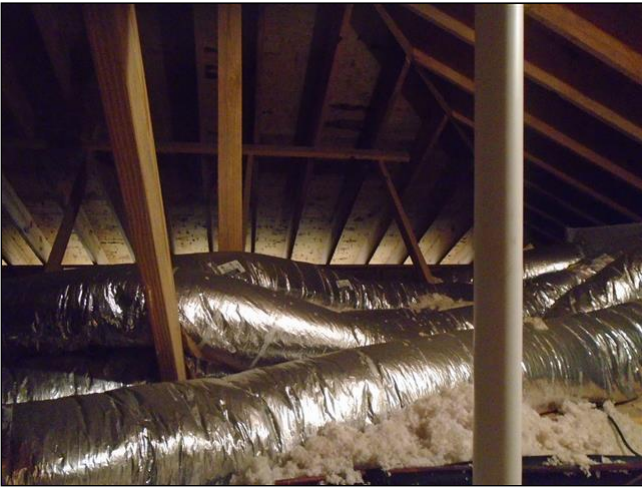
D. Item 1(Picture) Attic
