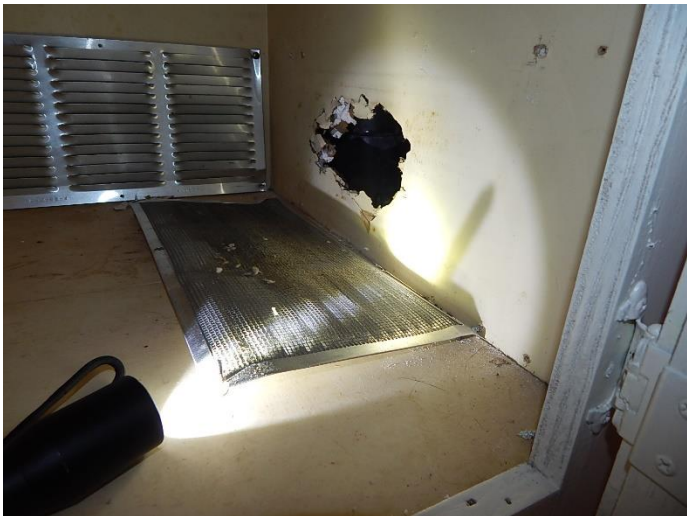
The tub access panels for the hall bathroom and master bathroom are in the hall bathroom lower cabinet (see above left photo). The opening on the right side of this provides visual access to the area below the hall shower/tub. In the above right photo, mold growth was visible on the framing boards for the hall shower/tub where it backs up to the wall behind the master toilet.
