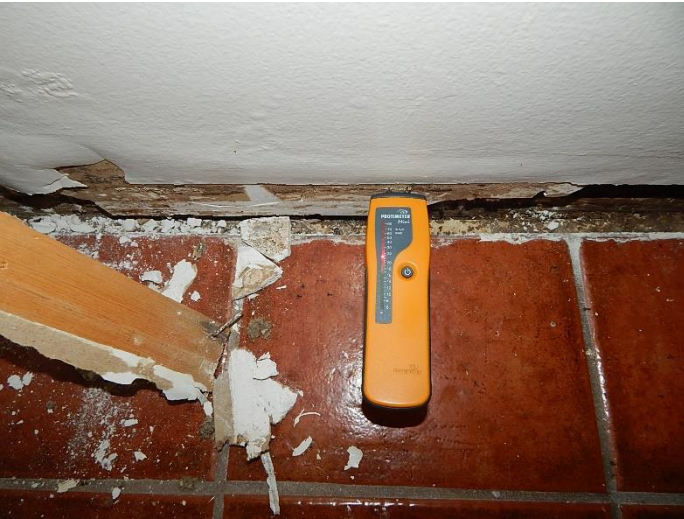
Moisture elevation and mold growth were observed on the exterior wall of the master bathroom.
