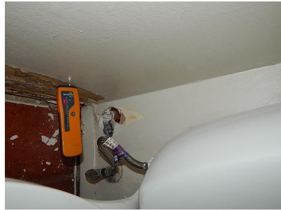
Moisture elevation and mold growth were observed on the exterior wall of the master bathroom.
