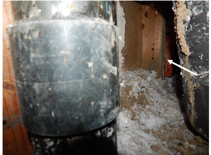
The tub access panels for the hall bathroom and master bathroom are in the hall bathroom lower cabinet (see above left photo). The opening on the right side of this provides visual access to the area below the hall shower/tub. In the above right photo, mold growth was visible on the framing boards for the hall shower/tub where it backs up to the wall behind the master toilet.
