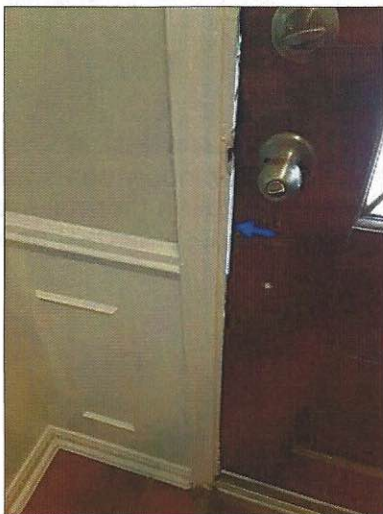
-There is visible light noted around the door. Mainly at - front door
