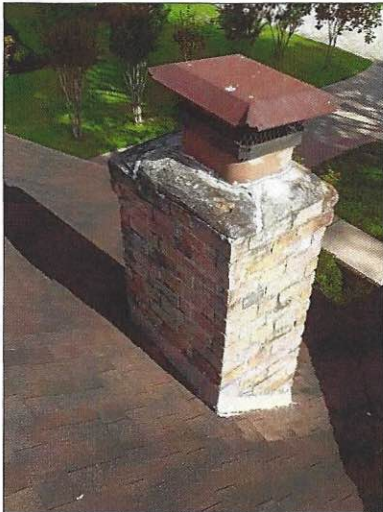
Overview of chimney
