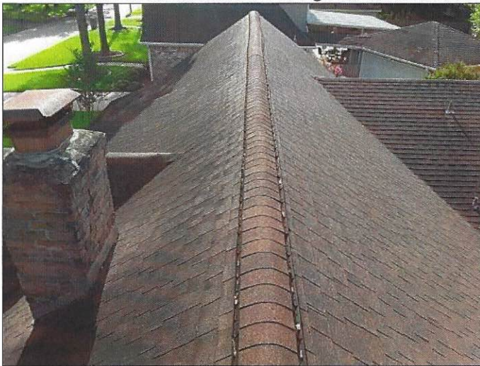
Overview of roof
