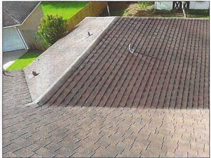
Overview of roof
