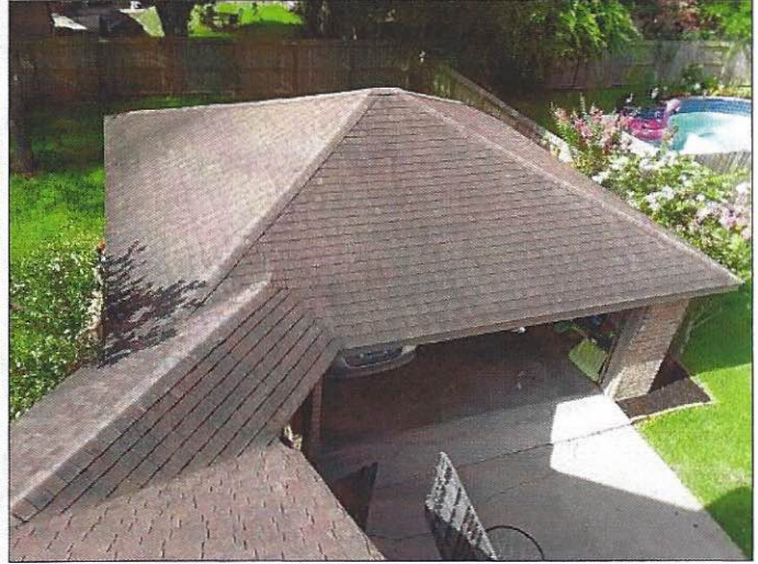
Overview of roof
