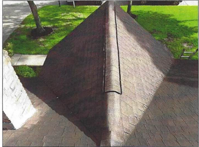
Overview of roof
