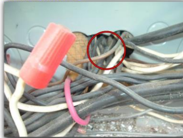
The protective wire grommet is missing.
