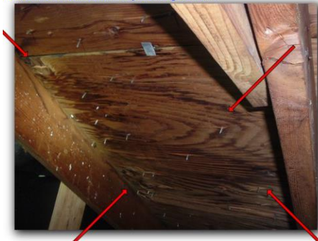
There is evidence of roof leaks/decayed decking in the attic.
