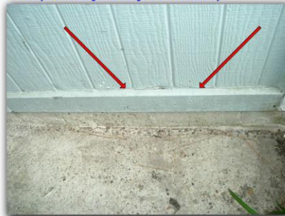
There is decayed wood siding/trim at the right area of the front entry.
