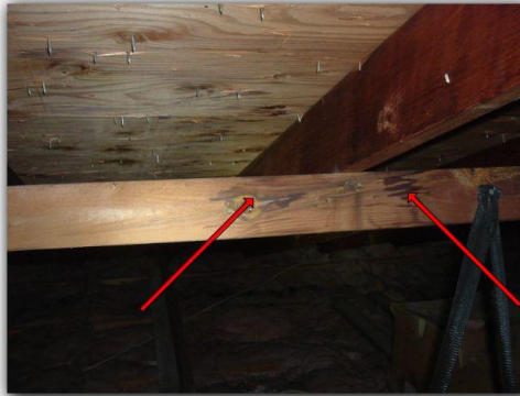
There is evidence of roof leaks/decayed decking in the attic.
