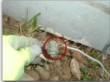
The ground wire is not connected to a ground rod.
