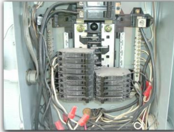
The protective wire grommet is missing.
