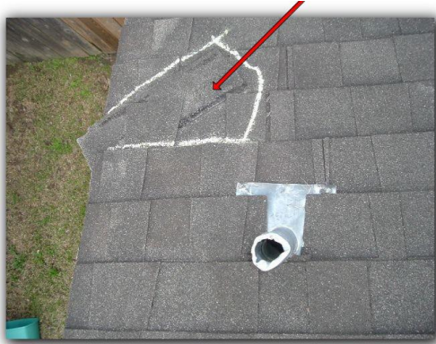
There is evidence of roof leaks/decayed decking in the attic.
