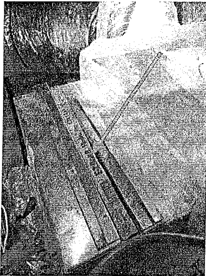
Filters are located by the heater in the attic space. The filter cover in the attic space is damaged
