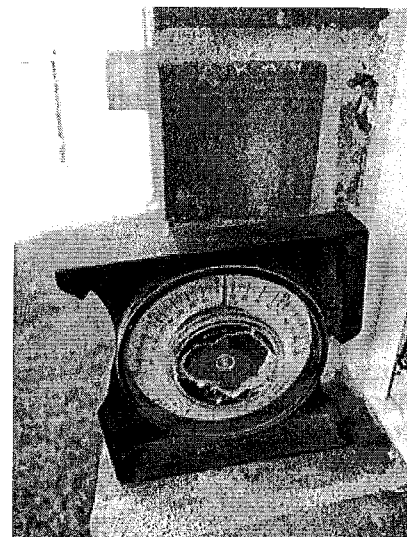
There are multiple locations around the house where the brick windowsill on the exterior do not have the proper slope. The windowsill should slope at a 15° angle away from the house.
