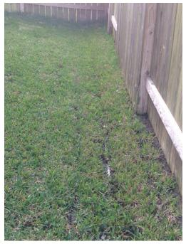
Runoff water from the roof discharges next to the house. We recommend the downspouts be routed sufficiently away from the structure to prevent puddling, pooling, and saturation of the soil around the building.
