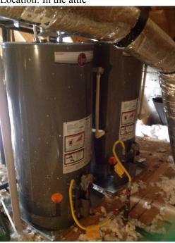
This is a newer water heater, was operating and with routine maintenance should be reliable for a number of years. However the insulation could block the drain.
