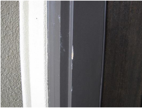
External luminaires not properly flashed/sealed.
