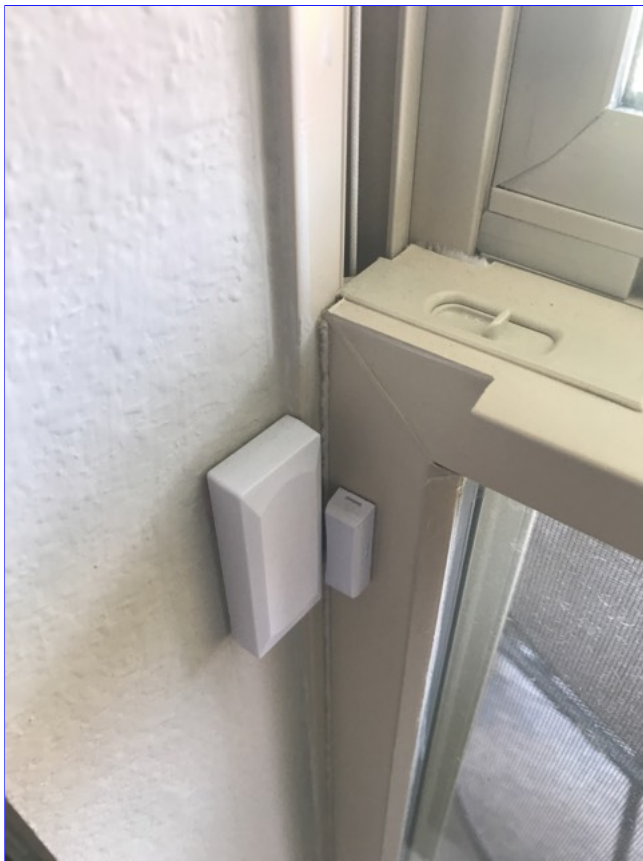
(2) Security sensors interfere with window opening.
