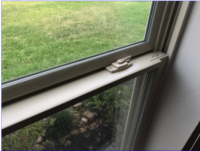
(2) Security sensors interfere with window opening.
