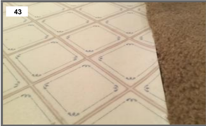
Master bathroom, vinyl flooring starting to come up where it meets the carpet.
