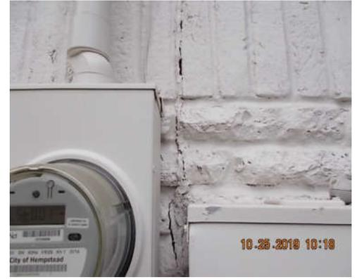
Brick veneer crack on south side of house.
