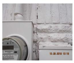
Brick veneer crack on south side of house.
