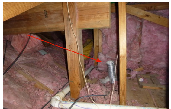
*Extend bath vents to the exterior
