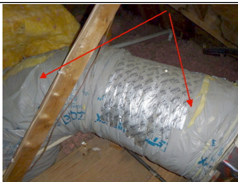
*Replace grey flex duct
