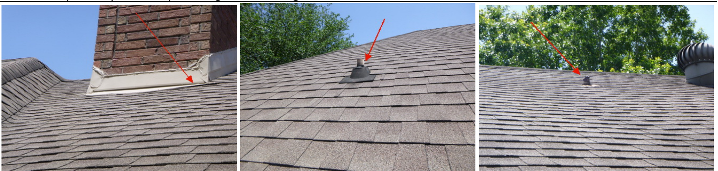
*Reset the chimney flashing
