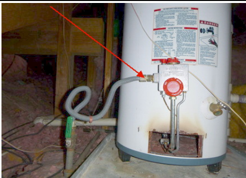
*Install a sediment trap
