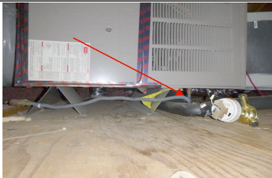
*Install a sediment trap
