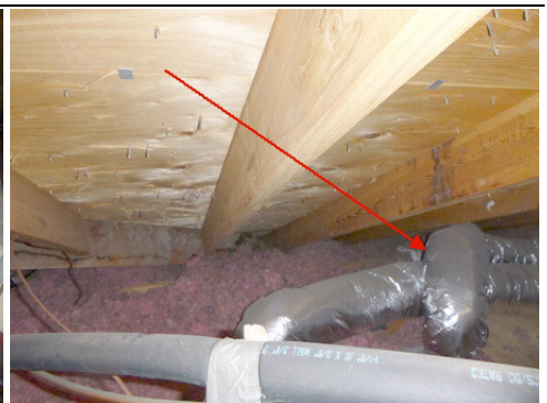
*Separate the flex ducting
