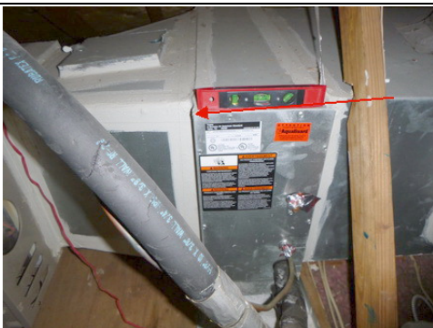
*Adjust the slope of the evaporator / p-drain pan; install a p-trap in the drain line at the evaporator
