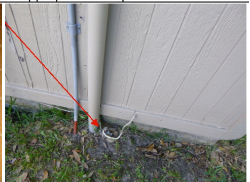
*Drive the ground rod fully into earth
