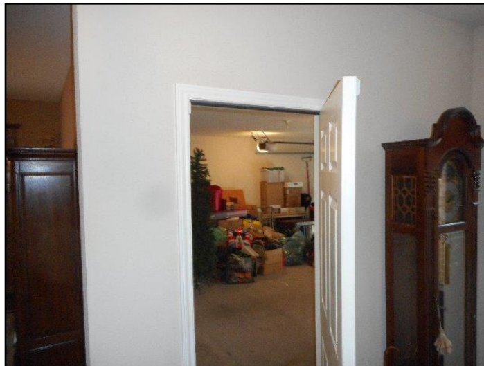
Self closing hinges do not shut door
