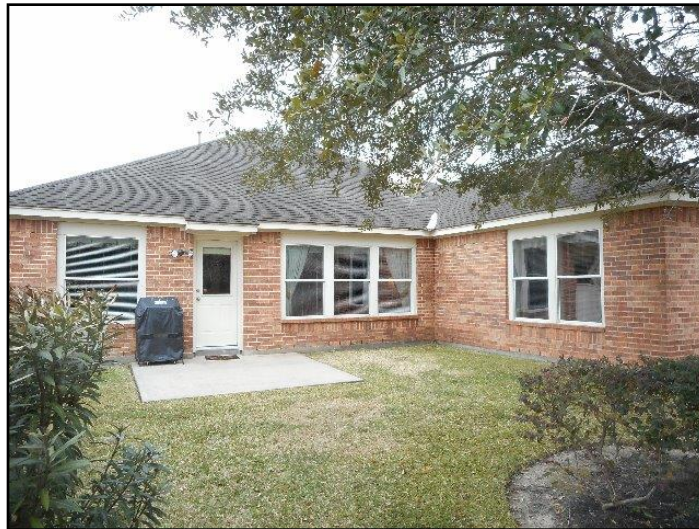
General view of exterior of home.
