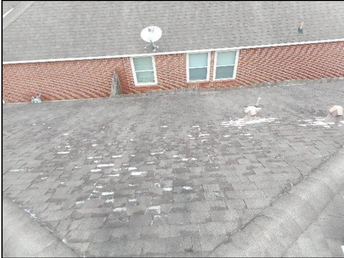
General view of roof covering.
