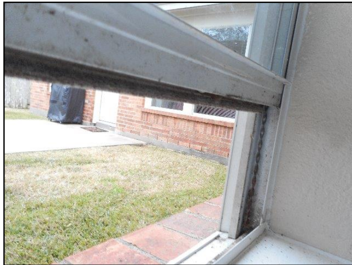
Detached window guide spring/balance
