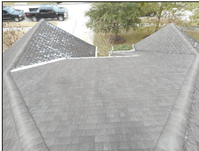
General view of roof covering.
