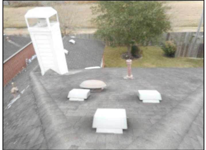
General view of roof covering.
