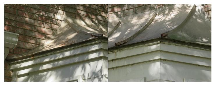
Kick-out flashing is required at the lower run of rain gutters to divert water away from the wall at the rain gutter/end of the roof.
