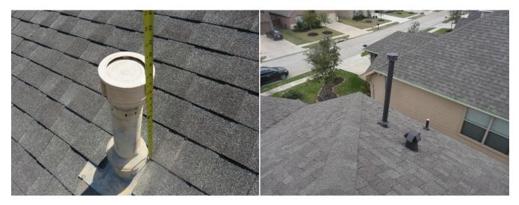
The exhaust flue/pipe exiting through the attic/roof of the home was resting directly against/too close to the combustible lumber of the roof sheathing. To prevent a combustion condition, this flue/pipe should be repositioned.
