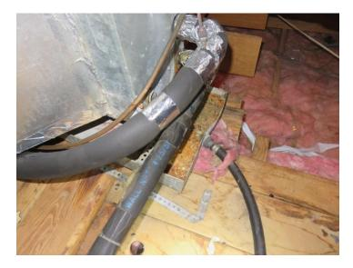
AC evaporator coil overflow pan shall be equipped with a water detection device in the primary drain line that will shut off the equipment should the drain line be blocked. (IRC M1411.3.1). It is recommended that the evaporator coil condensate auxiliary drip pan(s) be equipped with a safety floatswitch sensor that will shut-off the AC equipment in the event condensate enters the pan.
