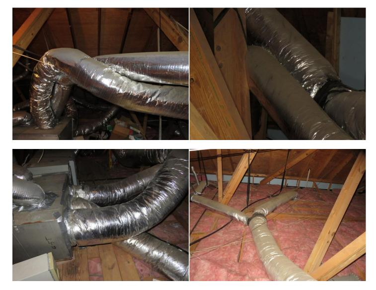
Some ductwork displays taping at plenums and some display bends/kinks.
