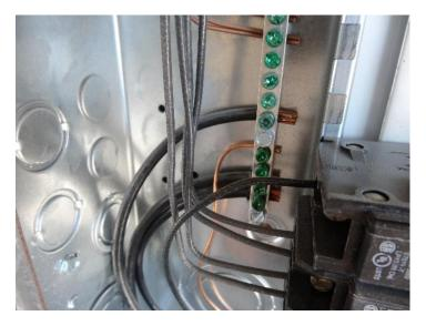
The ground and neutral bar, required to be in contact with the panel, do not appear to be. Normally a green grounding screw inserted in the bar at the top through the hole provided is present.
