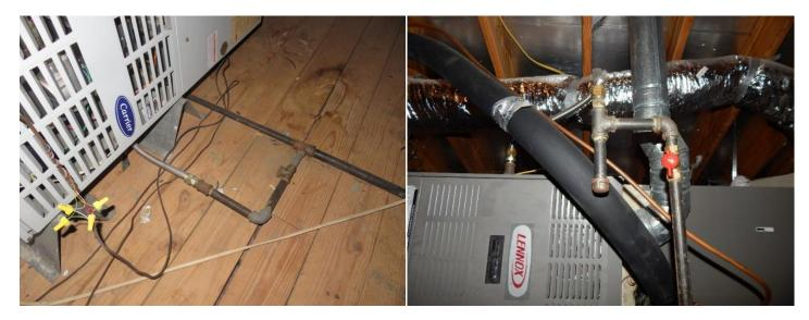
Hard, black pipe used to connect flexible steel natural gas pipe to the burner should protrude by approximately 2" outside the housing of the furnace appliance. Flexible tubing should not enter the housing of the appliance for connection to the burner.
