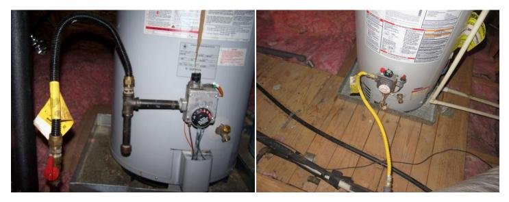
> The natural gas line for the appliance(s) is required to be secured within 12" of the shut-off valve.
