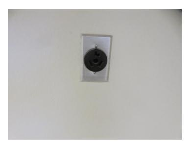
Closet lighting displays unprotected/incandescent bulbs that are unprotected by a globe. Should combustible storage be placed within 12" of one of the bulbs, a fire could ensue. These lighting fixtures should be replaced by fixtures having a globe surrounding the bulb.
