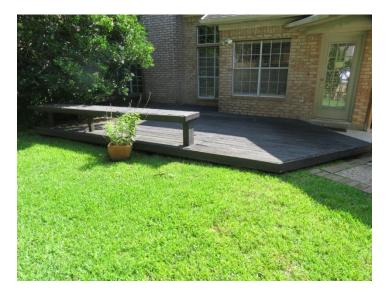
> The deck is of equal height as the foundation weep holes which could cause water to flow into the weep holes affecting the interior of the home.
