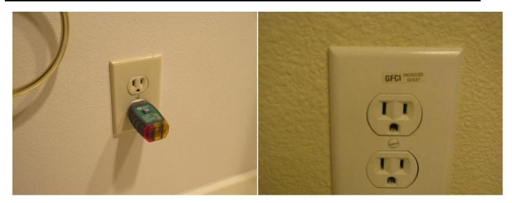
An outlet (GFCI) is a required installation at the exterior walls of the left side porch and atrium off the Master bathroom.
