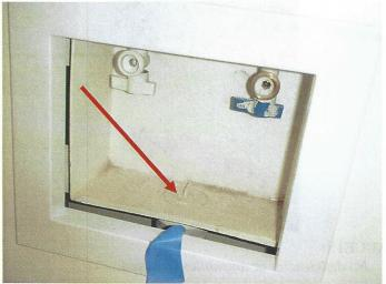
Water tight box knock out for washing machine drain line and gas line have large voids between boxes and wall.
