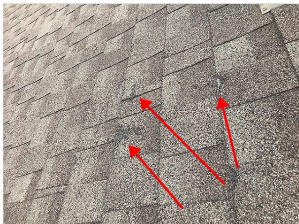
Damaged shingles
