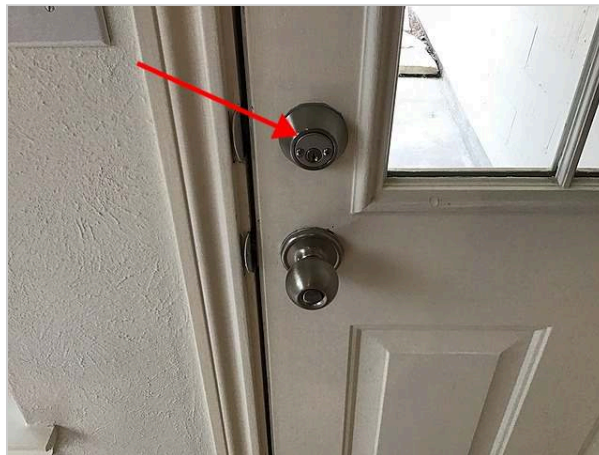
Keyed on the inside (rear exterior door)
