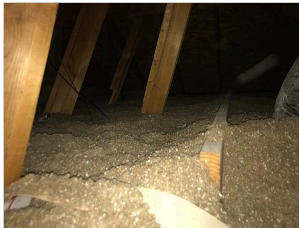
Blown insulation (approximately 8-10 inches)
