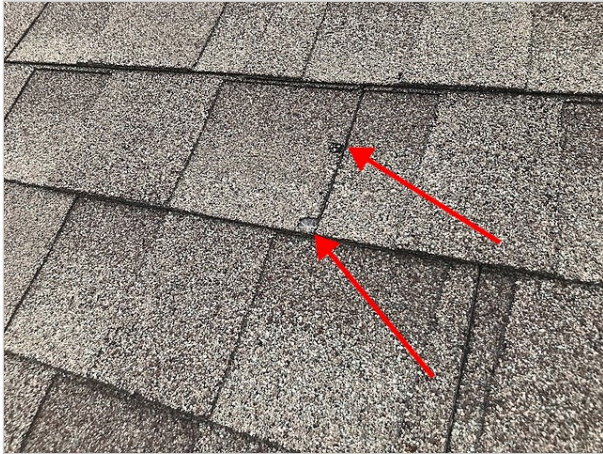
Damaged shingle
