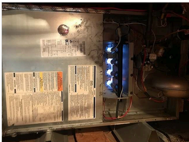
Burners viewed for inspection
