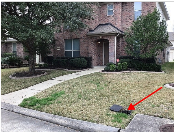
Water meter location
