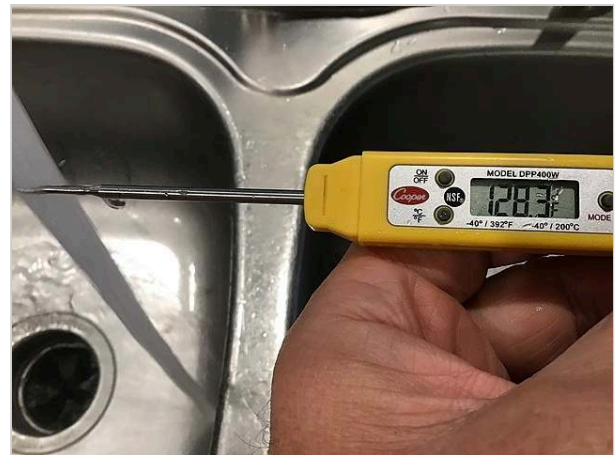
Hot water temperature at the kitchen sink (128.3 degrees)
