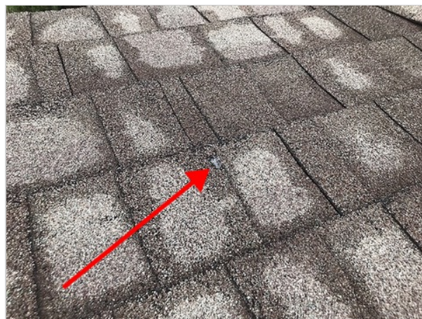
Damaged shingle
