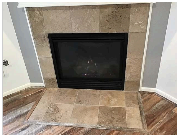
Gas lit for inspection
