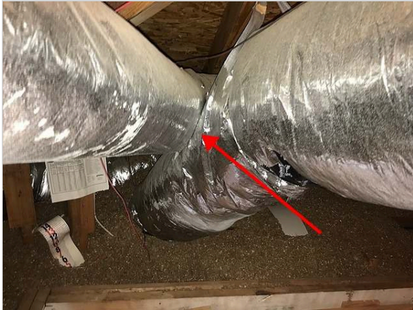
In contact with other duct
