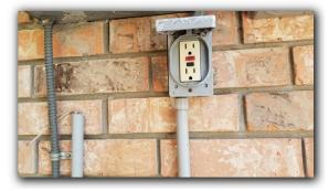
Not all receptacles at home were GFCI protected where currently required (all that can serve kitchen countertops, all at garage interior, exterior, dishwasher, pool house interior, and laundry room). Recommend installing GFCI protected receptacles as per current electric code at all receptacles in kitchen at counter tops, bathrooms, bars, exterior, utility/laundry rooms (adopted in 2014), dishwasher (adopted in 2014), all at exterior of home, and all in garage for safety.
