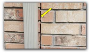
Install weep holes, required since 1992, at brick above lintels at maximum of 33" spacing above windows, entrance / exit jambs, garage overhead door jambs and elsewhere where lintels noted. Weep holes are also needed at lower course of bricks at exterior brick columns.
