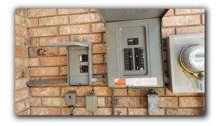
AFCI breakers are not noted at all living areas where required, per current electrical code, however these were not required when home was built.
