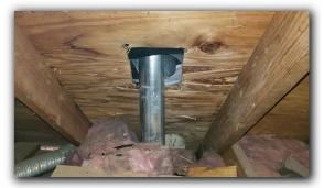
A flex line is improperly installed at temperature and pressure valve drain line. Properly reinstall <sup>3</sup>/<sub>4</sub>" CPVC, copper, or other approved smooth material at temperature and pressure line from temperature and pressure valve removed through wall to exterior with a non-threaded elbow within 6" to 2' above grade or other approved termination.
