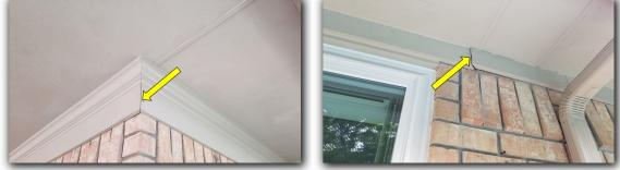
Mortar/stair step cracks and/or voids noted at multiple areas around brick exterior. Theses appear to be cosmetic and not structural in nature and can be repointed if buyer desires.
