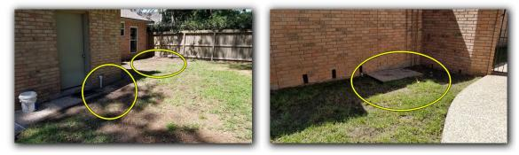
French drains noted at backyard and courtyard. Recommend buyer monitor these drains to ensure proper drainage during or after rainfall. Properly clean al drain basins (courtyard) and/or properly secure/replace loose or damaged grates, as needed.
