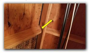
Adjust/repair or replace garage attic ladder at spring/hinge to close tight and securely at frame.
