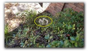
Missing and/or broken head noted at station 1.
