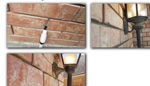
Seal and paint exterior siding/trim at nail heads, overlap edges, butt joints, separations, vertical joints.... etc. to prevent water penetration at dings, scuffs and holes to extend life.
