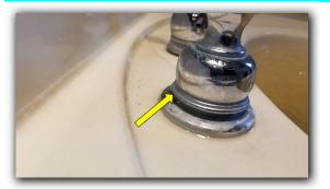
Anti-siphon valves are not noted at bibs; need to be installed.
