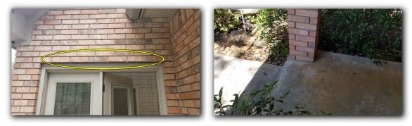
Area of minor deterioration is noted at south side of exterior trim/fascia. All deteriorated areas should be properly repaired and sealed, as needed, to prevent moisture penetration.
