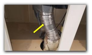
East exterior vent termination is noted as damaged and is in need of repair/replacement.
