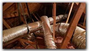
Double filtering (filters at returns and at media filter housing in attic) reduces airflow, reduces life and efficiency of compressor, as well as cooling of house and increases cost of operation. Recommend removing return grate filters throughout home or media filter at system in attic.
