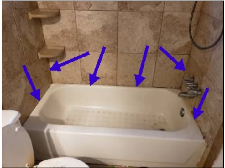
-Recommend sealing the tub/shower surround to help prevent water penetration to underlying materials. Mainly at - hall bath
