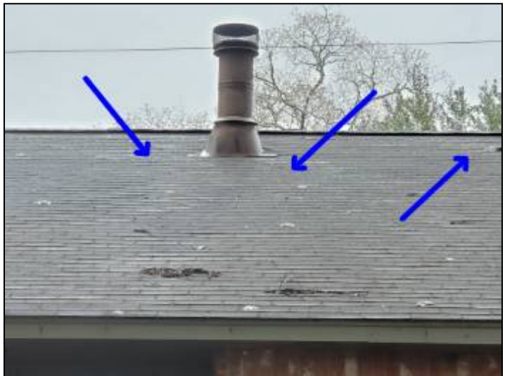
-Due to the excessive granular loss on the roof covering the roof may age prematurely. We recommend further review of the roof system for a better understanding of the present condition.
