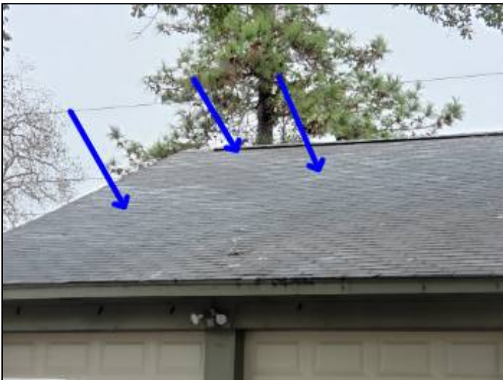
-Due to the excessive granular loss on the roof covering the roof may age prematurely. We recommend further review of the roof system for a better understanding of the present condition.
