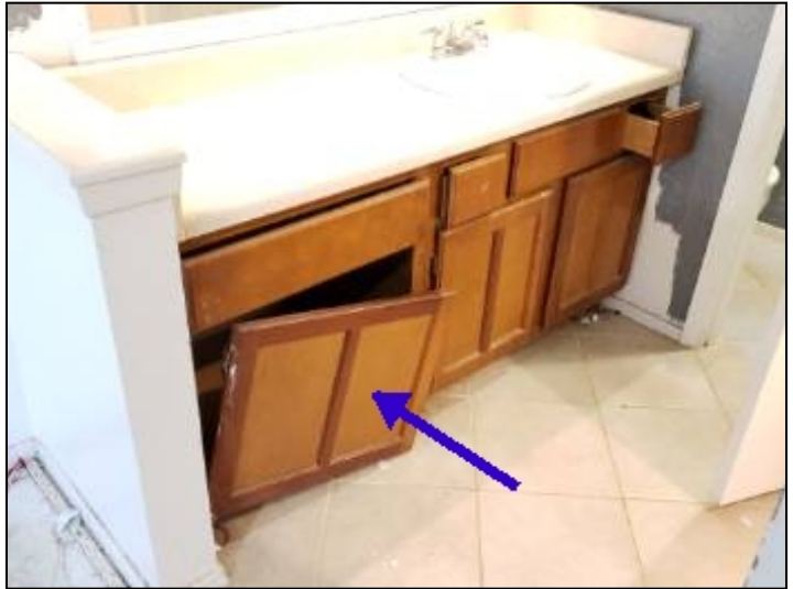
-Although cabinets are not inspected it was noted that cabinets are damaged throughout.
