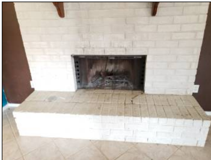
Overview of fireplace
