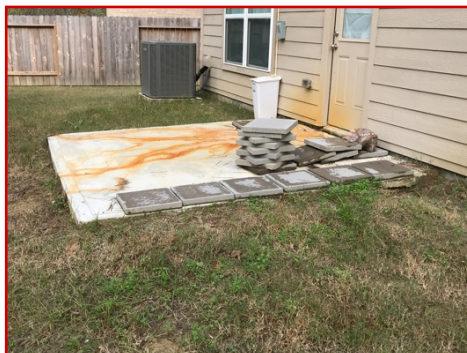
Patio slab in rear, ok, no cover
