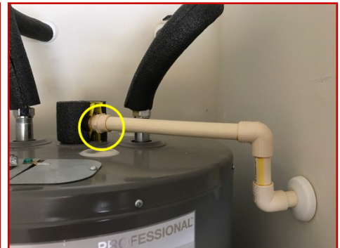
Coupler should be Metal
