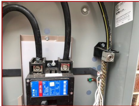
Aluminum mains with anti oxidant present
