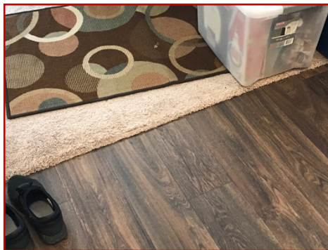
Carpet tacks can be felt in the seam between the living room and dining room
