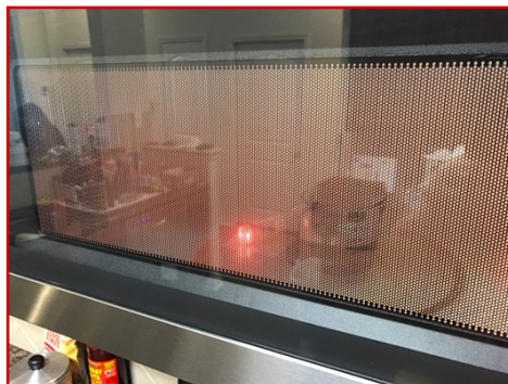
Microwave detector showing unit functioning properly
