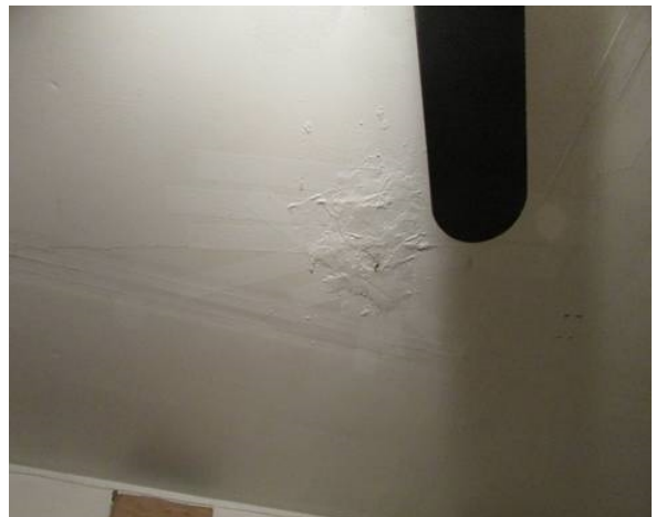
Repair ceiling - kitchen
