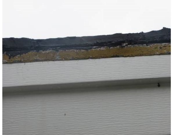
Damaged drip edge and shingles - near side walk
