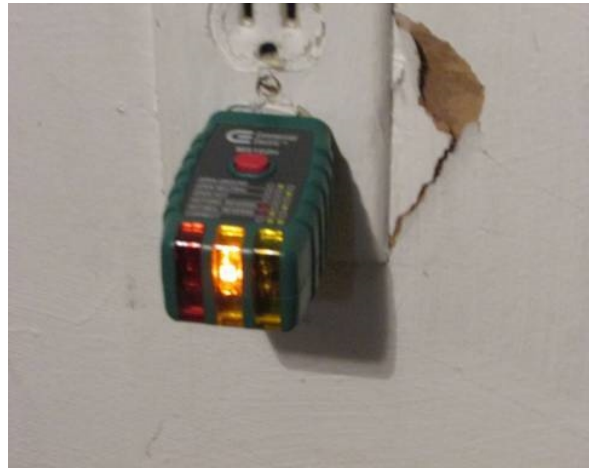
Open ground - interior
