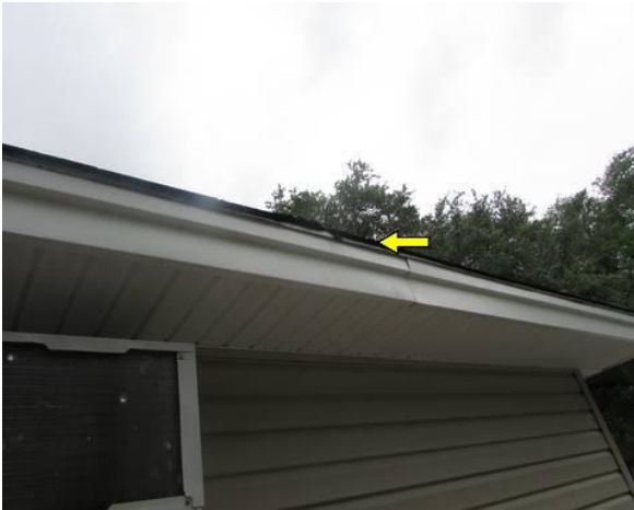
Damaged Shingle
