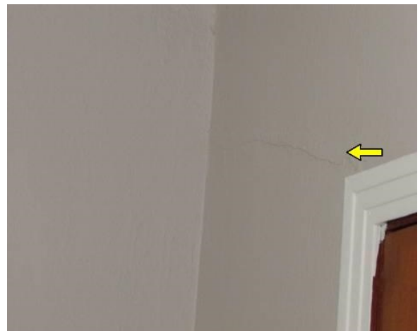
Wall crack
