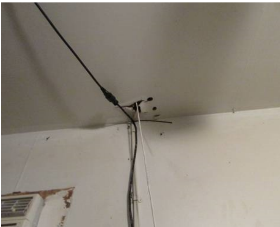
Repair holes - garage
