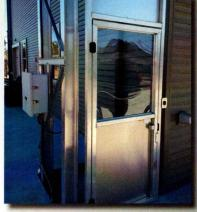
Self-closing doors and gates are equipped with safety interlocks to keep doors locked when the lift is away from the floor level.
