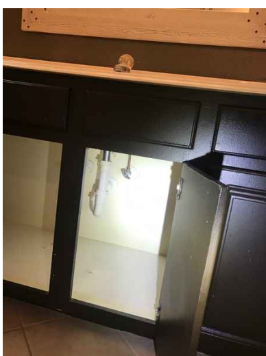
General Photos of Gas Meter(s):
