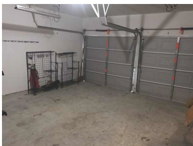
General Photos of Structure:
