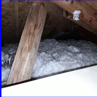
Attic insulation blown
