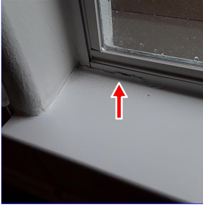
E. Item 1(Picture) Areas at some window sill trim, need fresh caulk
