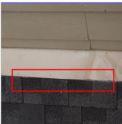
C. Item 1(Picture) First level roof system at rear
