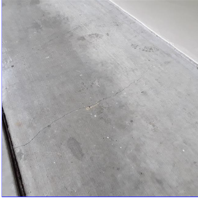
L. Item 1(Picture) Driveway at garage door
