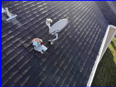
Roof surface is Architectural Shingles (30 year)
