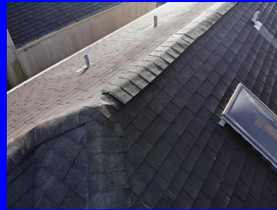
Roof surface is Architectural shingles
