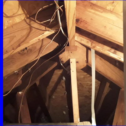
Attic framing rafters and decking
