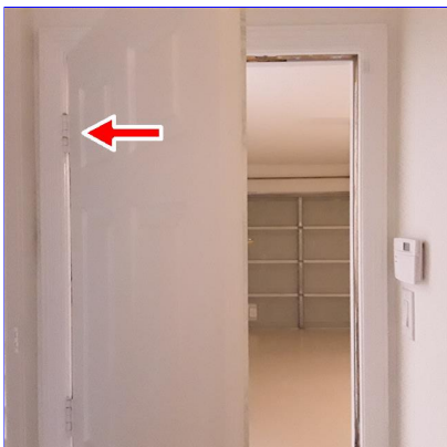
G. Item 1(Picture) Should be self closing hinge
