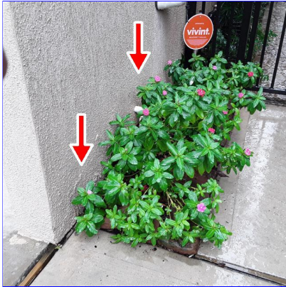
A. Item 1(Picture) Right side front of home at entry
