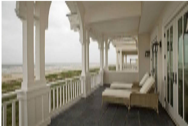
Figure 14 - Porch with columns, brackets & guard
