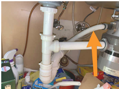
Kitchen under sink
