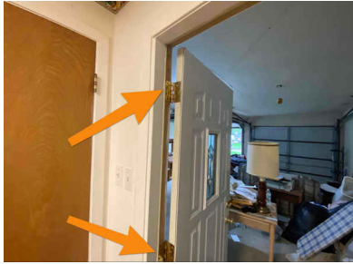
Door leading to garage
