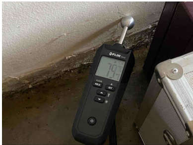
Right wall in garage
