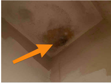
Secondary bathroom linen closet ceiling
