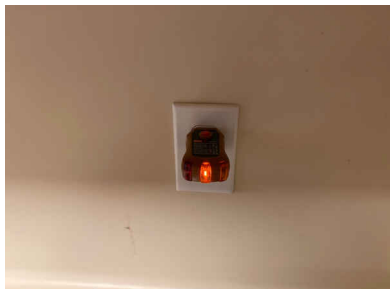
Kitchen right of sink
