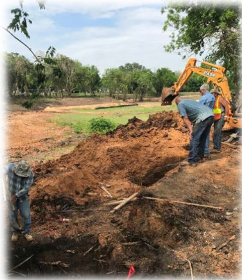
Wessendorff Trail Construction – Summer 2017
