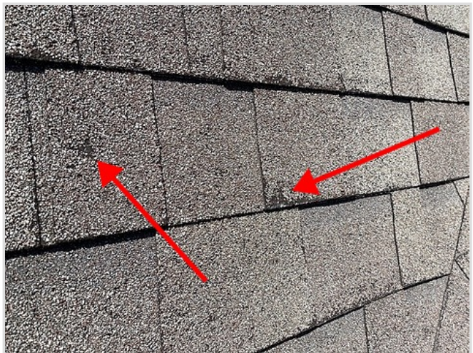
Damaged shingles
