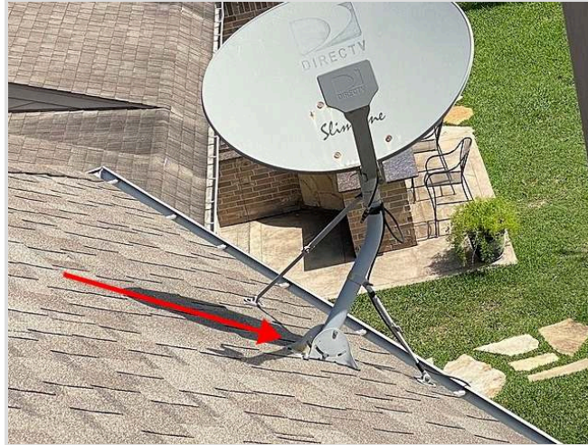
Installed over shingles
