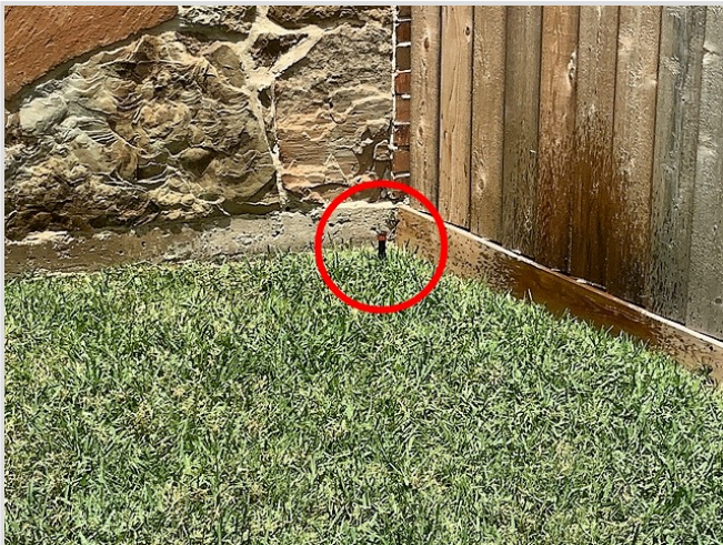
Improper spray pattern
