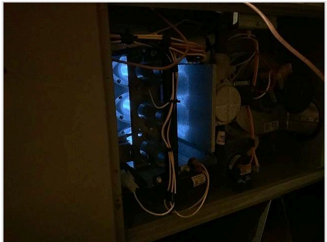
Burners viewed for inspection (second floor unit)
