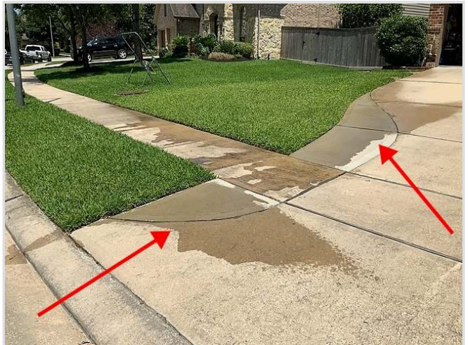
Improper spray patterns
