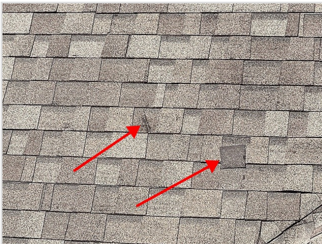
Damaged shingles
