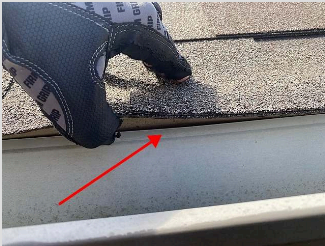
Installed in front of the drip edge
