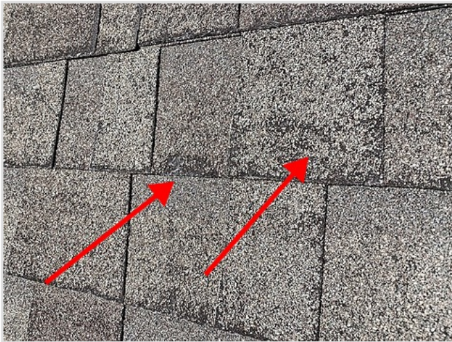
Damaged shingles
