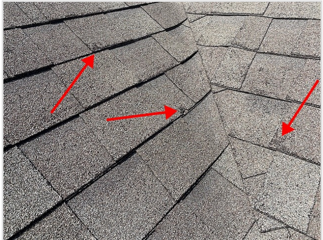
Damaged shingles
