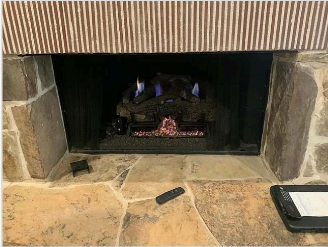
Performing as intended (interior fireplace)
