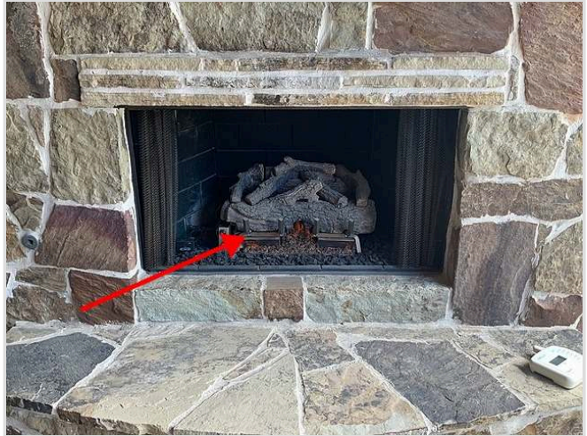
Performing as intended (exterior fireplace)
