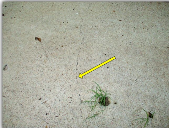
Crack in back porch.
