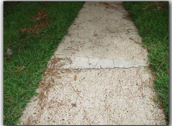
Front side walk has heaving of slabs causing tripping hazards.
