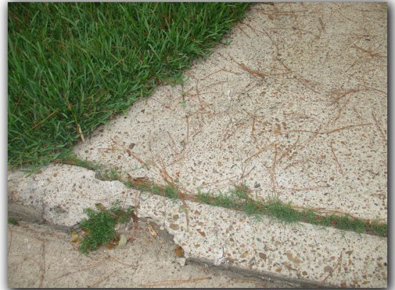
Front side walk has heaving of slabs causing tripping hazards.
