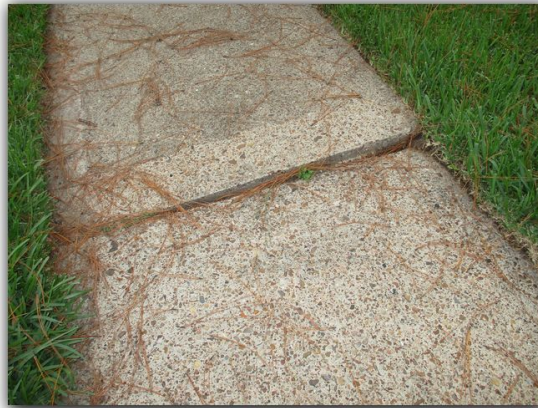
Crack in back porch.
