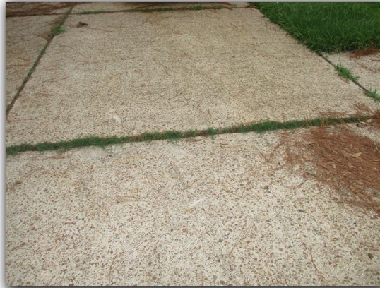
Front side walk has heaving of slabs causing tripping hazards.
