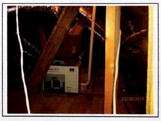
Clean all insulation and debris from the mechanical drain pan under the air handler and water heater. The present condition may create the pans to overflow if water leaks should occur from the unit.
