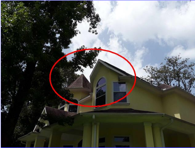
C. Item 17(Picture) front of roof
