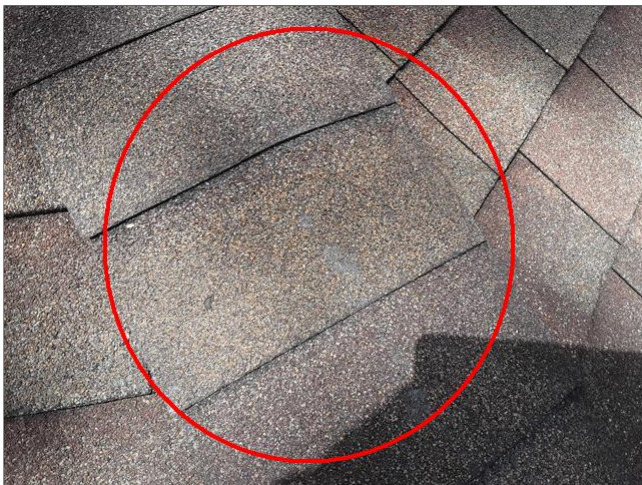
C. Item 9(Picture) front of roof
