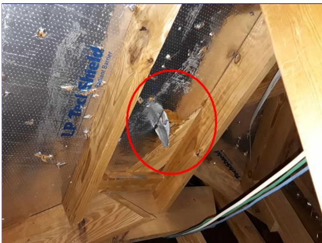
D. Item 3(Picture) attic
