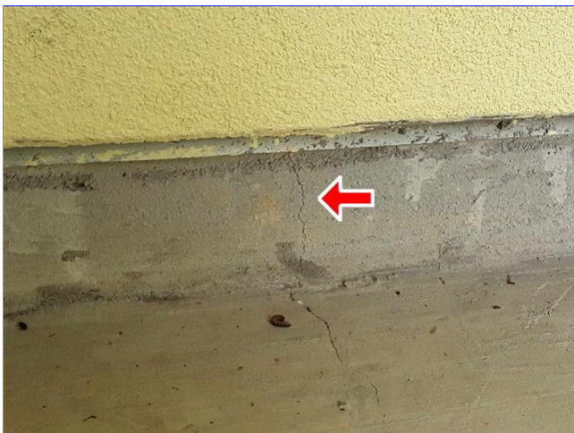
A. Item 1(Picture) rear of home
