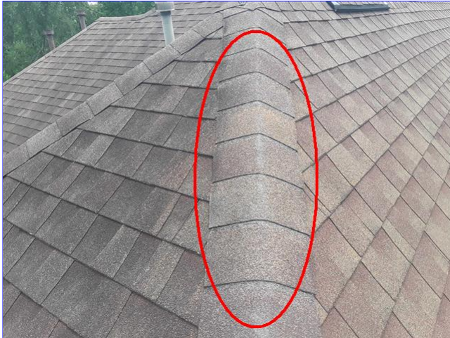
C. Item 12(Picture) rear of roof
