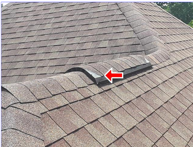
C. Item 13(Picture) rear of roof
