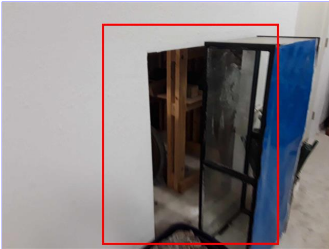
L. Item 7(Picture) multiple areas of garage
