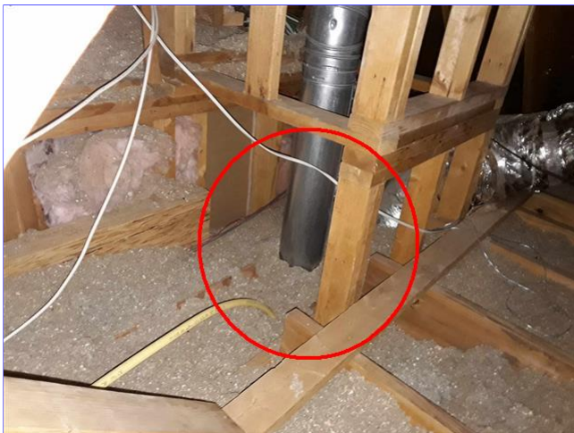
D. Item 2(Picture) attic
