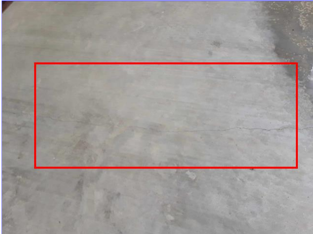
K. Item 1(Picture) rear of home
