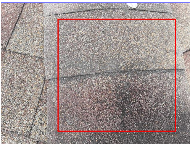
C. Item 10(Picture) front of roof
