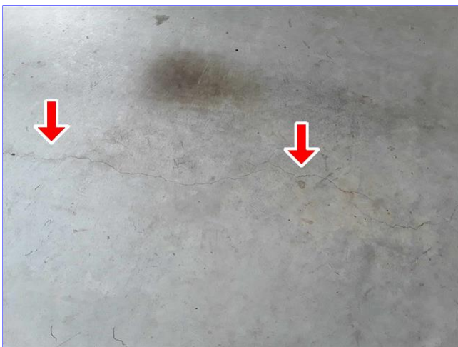
F. Item 1(Picture) garage
