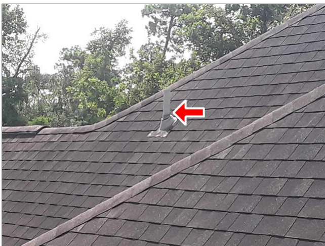
C. Item 15(Picture) front of roof
