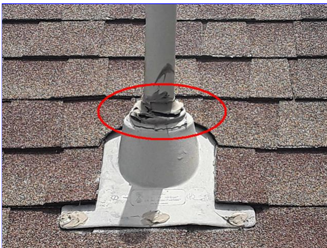
C. Item 16(Picture) rear of home
