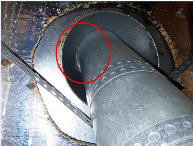
D. Item 1(Picture) attic
