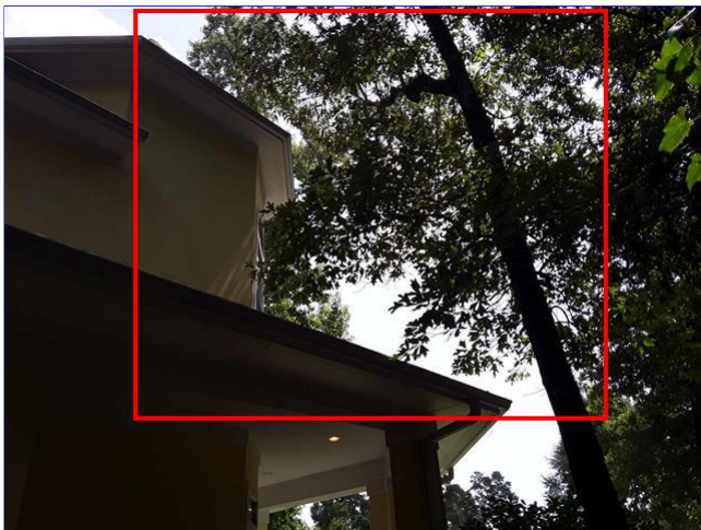
C. Item 8(Picture) front of home
