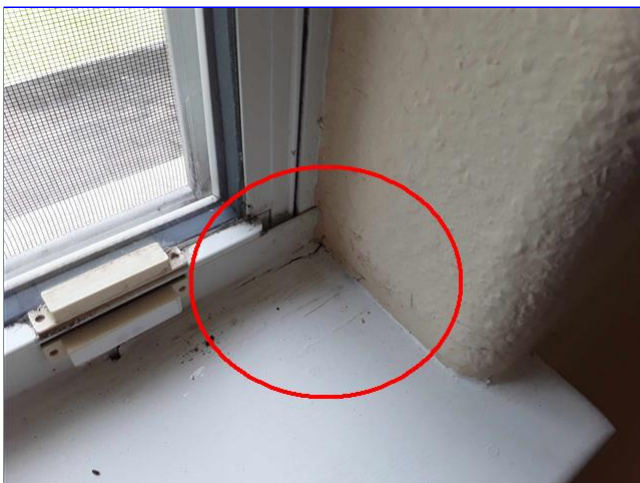
E. Item 20(Picture) front upstairs guest room
