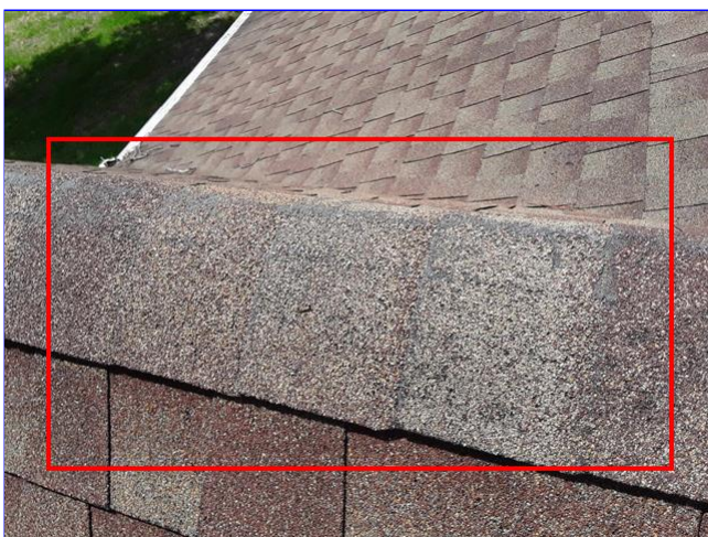
C. Item 11(Picture) front of home
