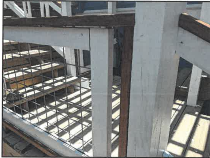
40. Spindles (balusters) climbable
