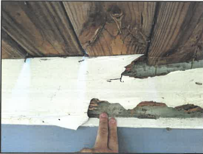
28. Rot or insect damage
