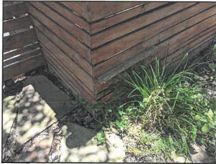
42. Rot or insect damage
