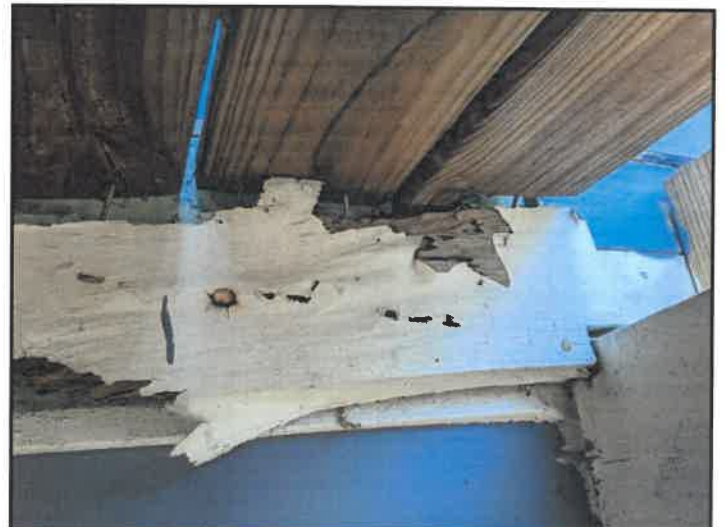
31. Rot or insect damage
