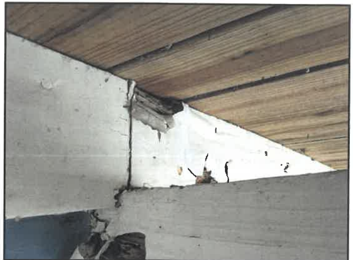
29. Rot or insect damage
