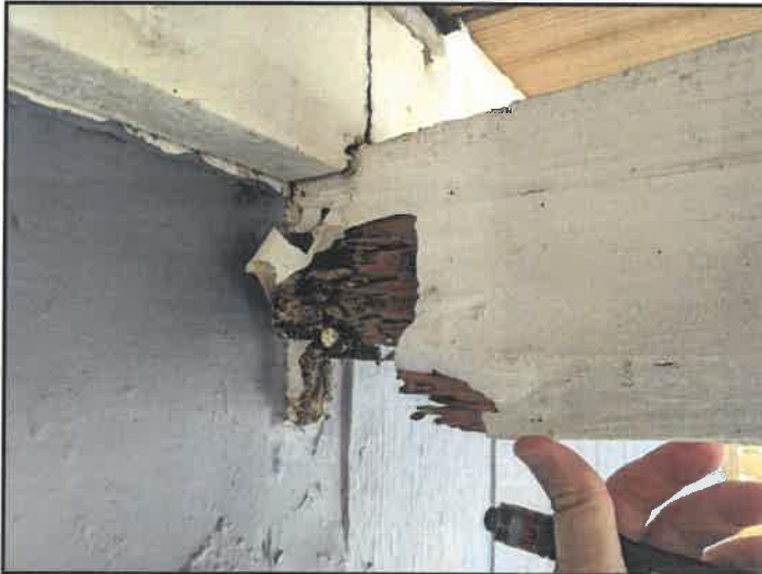
30. Rot or insect damage
