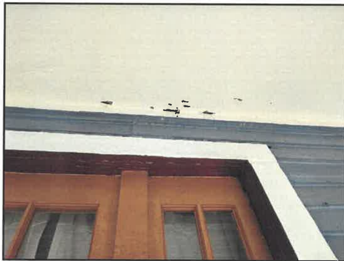
41. Rot or insect damage
