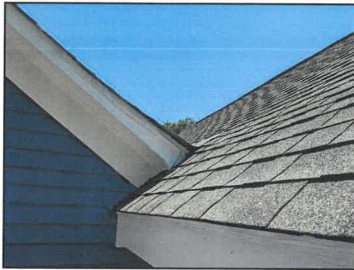
1. Asphalt shingles
