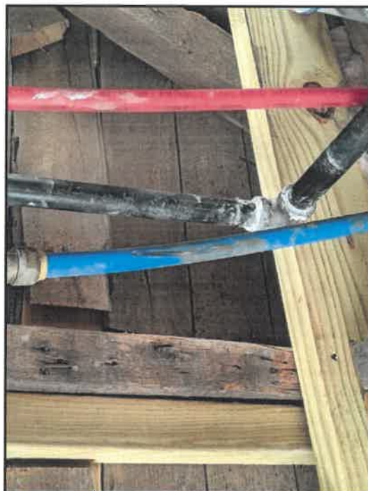
85. Inadequate support
