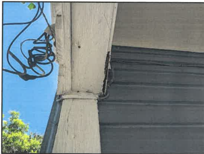
27. Rot or insect damage
