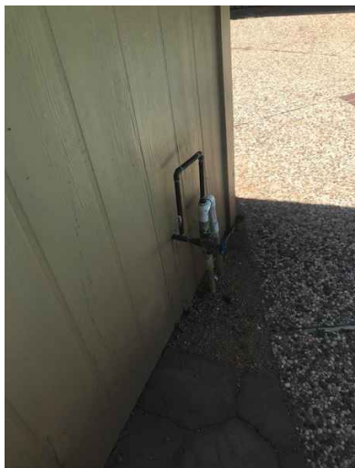
Filtering Components:: Skimmer
