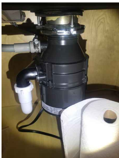
General Photos of Range Hood/Exhaust Systems:
