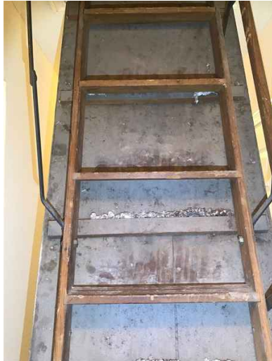
Type of Attic/Roof Ventillation: Soffit vent, Gable vent
