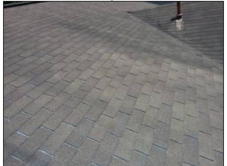
Overview of roof
