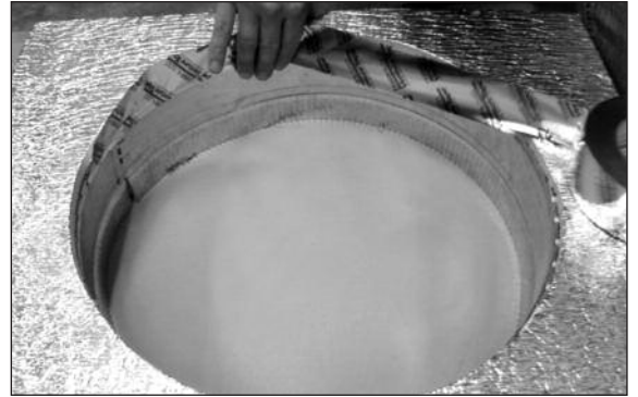
10. Put the insulation to the inner side of the panel and fix the insulation to the collar with a duct tape.
