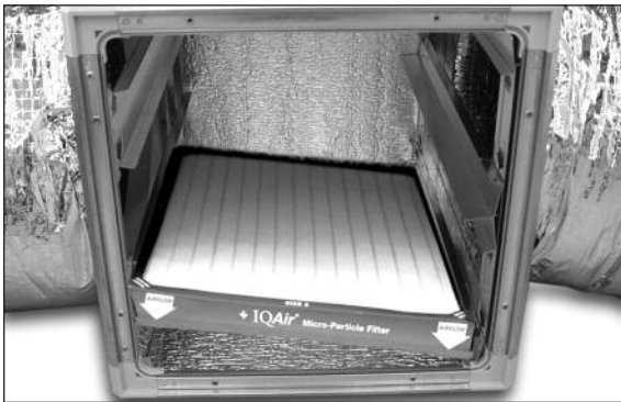
5. Insert new filters starting from the bottom.
