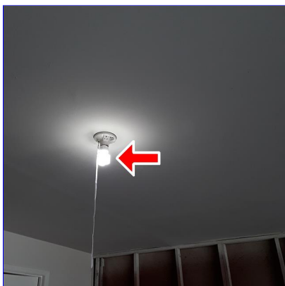
B. Item 2(Picture) garage
