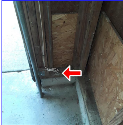
B. Item 9(Picture) garage
