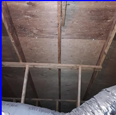
stick built roof structure
