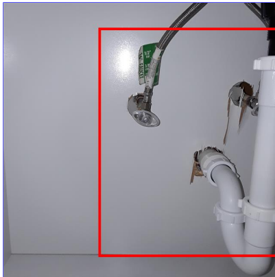
E. Item 16(Picture) primary bath
