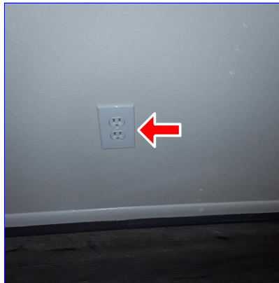
B. Item 25(Picture) multiple outlets
