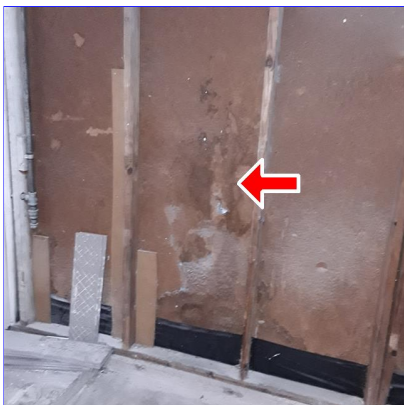
E. Item 22(Picture) garage right
