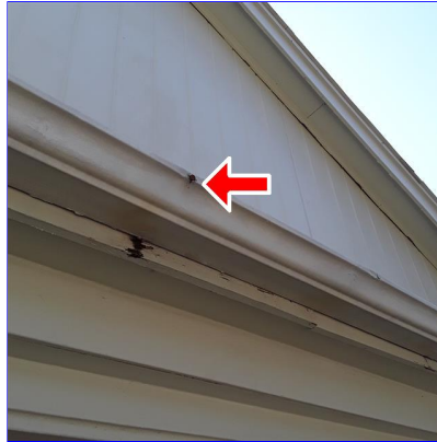
B. Item 2(Picture) garage
