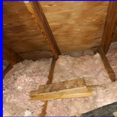
batt insulation less than 6 inches
