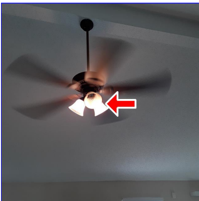
B. Item 20(Picture) multiple areas
