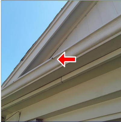
B. Item 1(Picture) garage
