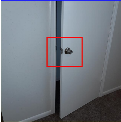
G. Item 8(Picture) front bedroom
