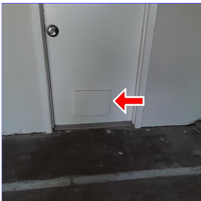
G. Item 1(Picture) garage
