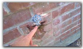
• The hose bib located on the front of the home leaks when in the closed position.
