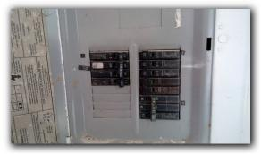
• Breakers were found in the off position upon inspection. With no knowledge as to why the breakers were off, the breakers were not engaged. Engaging a fault tripped breaker can potentially cause damage to the circuit or devices plugged into the circuit. This should be evaluated by a licensed electrician.
