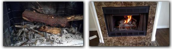
• The fireplace contains a gas log / starter arrangement and a chimney damper that is not blocked in the open position. The damper must be blocked open to ensure combustion byproducts from a gas fire to exit the house via the chimney.
