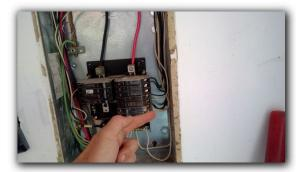
• A 40 amp breaker is lugged into wiring much smaller than the 8 awg copper wire it is rated for. As a result, this circuit is over-fused and not properly protected. This should be corrected by a licensed electrician.
