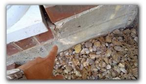
• The foundation's rebar is visible at the edge of the garage foundation and should be properly sealed to prevent deterioration.
