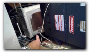
• The furnace exhaust vent flue is too close to combustibles. A "B-vent" requires 1 inch of clearance. Single wall vent flues require 6 inches of clearance.
