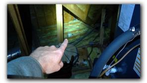
• Conduit is damaged/separated, exposing wiring outside the home. This should be repaired.
