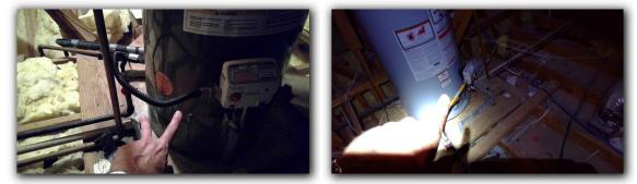
• The water heater exhaust vent fluesares too close to combustibles. B-vent flues require 1 inch of clearance. Single wall flues require 6" of clearance. The lack of clearance creates a potential fire hazard and should be corrected.
