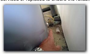
• There is no pressure gauge on the system. When water is turned on, the pressure switch turns on and off very quickly. This causes system pressure to greatly fluctuate. This is also very hard on the submersible pump. This well
