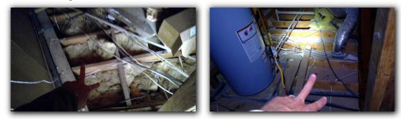
• The attic access door transitions from a conditioned space to the unconditioned attic. The door lacks weather stripping and insulation. This can result in heating and cooling losses.
