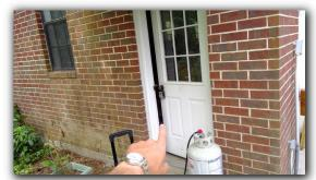
• Weather stripping is missing around exterior door(s). This can result in significant energy loss and potential moisture intrusion into the home.
