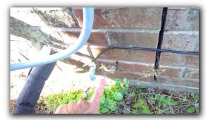
• The water temperature at faucets / showers was observed to be in excess of 120° F. Water above this temperature creates a burn hazard for its occupants. The water heater thermostat should be adjusted downward accordingly.
