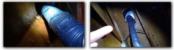
• The TPV drain line is not plumbed to the exterior or is not plumbed to within 6 inches of the garage floor or secondary drain pan. This creates a potential scalding hazard and water damage should the TPV be opened.
