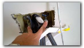
• A gas supply line is not in use and is uncapped. All gas supply lines should be capped when not in use for safety. In the event the gas valve is opened, the cap will prevent the structure from being filled with gas.
