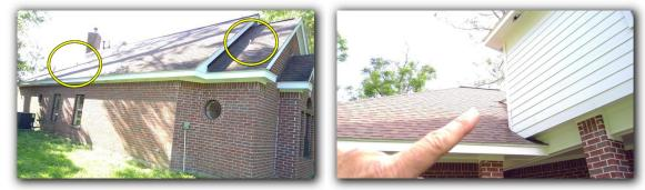
• Missing flashing was observed. This should be corrected to prevent wind driven rain and moisture intrusion into the roof system.
