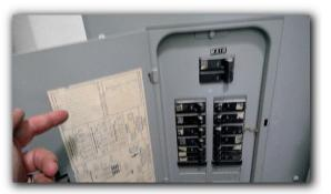
• White wires connected to breakers are not marked with red or black tape as an indicator they are "hot" conductors.
