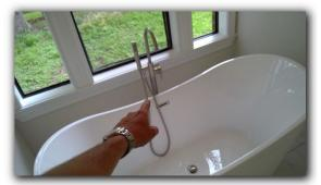
• The master shower is not draining at an adequate rate, indicating a potential blockage in the piping serving this fixture.
