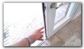
• French doors are present that do not latch/lock properly. Adjustment of the door/hardware is recommended.
