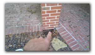
Note: Any area where the ground or grade does not slope away from the structure at least 6 inches per 10 feet is considered an area of improper drainage. Proper drainage and soil moisture content should be maintained around the foundation to minimize future foundation problems. Underground drainage systems are not inspected. They should be maintained for proper drainage.
