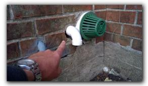
• Expansion joints are present in the brick/stone veneer walls that need to be resealed to prevent moisture intrusion into the wall system.
