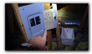
• One or more knockouts are missing, allowing for unsafe access into internal portions of the electrical panel.
