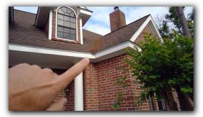
• Lead roof jacks are in need of replacement. In their present condition, moisture penetration in to the attic space is possible.
