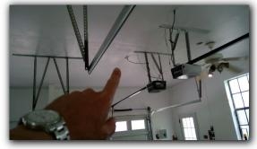
• Open ended wiring was identified that does not terminate in a junction box or fixture. This wiring should be further secured by a licensed electrician.
