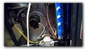
• A sediment trap is not present on the gas piping before it's entry into the furnace. A sediment trap is necessary to capture matter or debris in the gas line that could foul the gas valve or burner system. One should be added.
