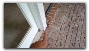
• There are penetrations present in exterior wall systems that should be sealed to prevent water intrusion into the home.
