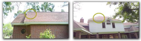
• Lifted flashing was observed. This should be corrected to prevent wind driven rain and moisture intrusion into the roof system.
