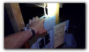
• The dead front panel is missing a screw or screws.
