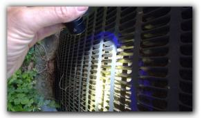
• The evaporator coil cabinet is severly rusted on one of the A/C units.
