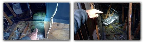
• The primary condensate line is not fully insulated. Without proper insulation, the cold water in the drain line can cause condensation to form on the piping that could drip and damage attic surfaces.
