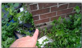
• Rusting rebar is showing through the surface of the garage slab. The slab is noticably damaged in areas.
