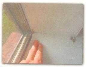
☑ Undetermined stained and/or damage areas were noted on the wall and/or trim areas next to second floor bathroom tubs. This damage areas are usually caused by moisture escaping the tub area during operation/use. Randomly tested these wall areas with a moisture meter. Moisture did not appear to be present at these areas at the time of inspection.
