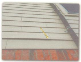
☑ The eve/soffit areas did not appear to be properly flashed and/or sealed where they butt up to the lower split level roof areas of the home. ☑ front ☑ rear ☑ left I was able to view daylight in some of these areas in the attic. These areas are commonly not properly sealed. (Should be properly sealed and/or flashed to prevent small animals/rodents from possibly entering the eve and possibly the attic area.)
