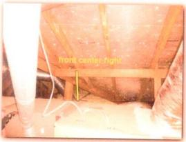
☑ Missing purlin and vertical purlin braces/supports noted at the attic area above the garage. This may or may not be part of the engineered design. (Engineer and engineered plans not present
