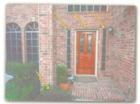
☑ Some rusting of the metal lintels were noted above one or more windows and/or doors. (The metal lintels, which support the brick veneer, should be sealed and painted to prevent damage to lintel and/or brick veneer.)
