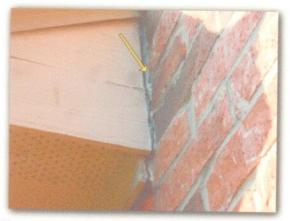
☑ The weep holes are missing at the bottom area of the brick veneer wall area above one or more window and/or doors and bottom of front column of the home.
