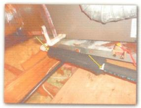
Air leaks at the evaporator housing.
