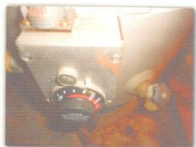
☑ The interior burner access cover was not properly secured - SAFETY HAZARD.
