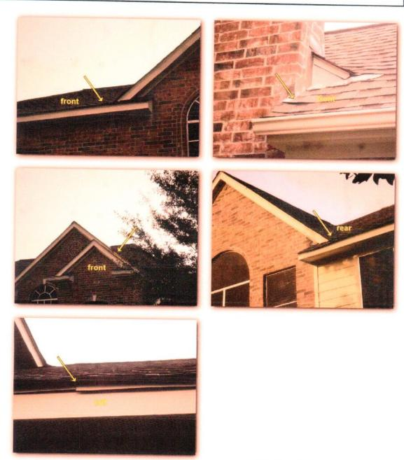
☑ There was no rain diverting roof/wall flashing installed at several rear locations. (Keeps excessive water run-off off the exterior walls of the home.) ☑ front
