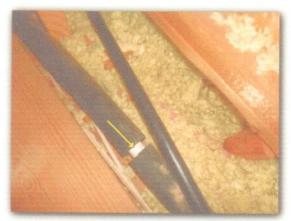
☑ Air leaks at the evaporator housing.
