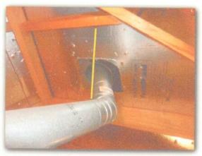
☑ The gas valve/line assembly is obstructing the heater's service access panel.
