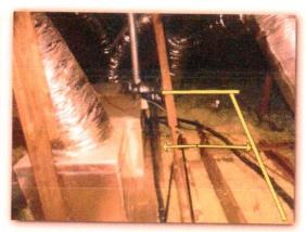
Attic Ventilation: ☑ Soffit Vents ☑ Ridge Vents ☑ The attic ventilation/insulation baffles are missing at one or more eve/soffit vent locations.
