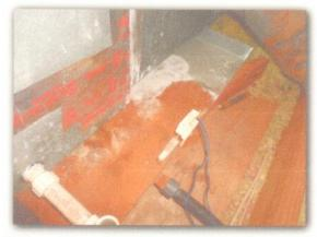
☑ The primary drain line needs insulation for full length of attic run.
