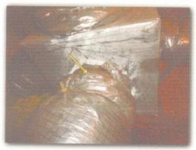
☑ Ducts touch each other or lay on the attic insulation at one or more locations. Ducts should not touch each other or lay directly on the insulation due to moisture/condensation.
