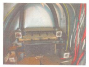
$\ensuremath{\,arphi\,}$  Neutral/white wires used as second hot is not re-identified (Black mark or black tape.) on 220 current. (common)
