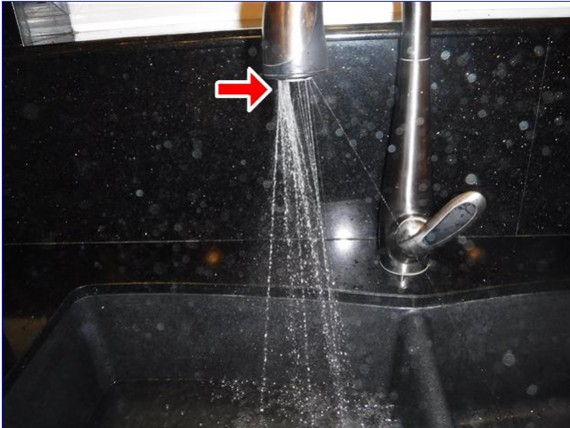
A. Item 3(Picture) Irregular spray pattern here
