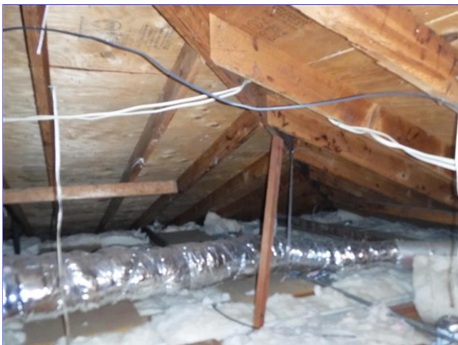
D. Item 1(Picture) Roof structure view.
