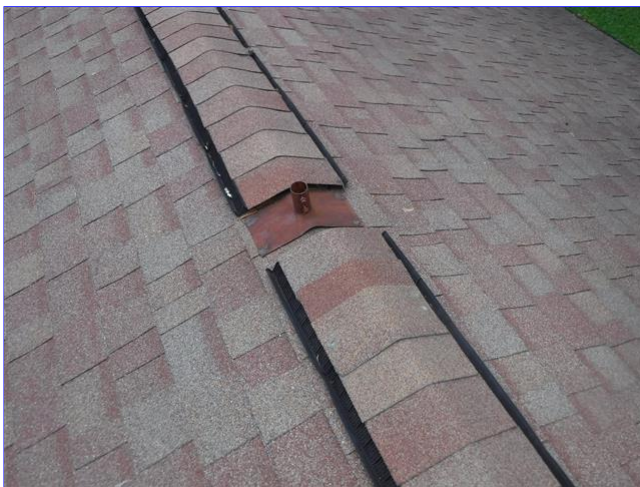
C. Item 4(Picture) View of roof.
