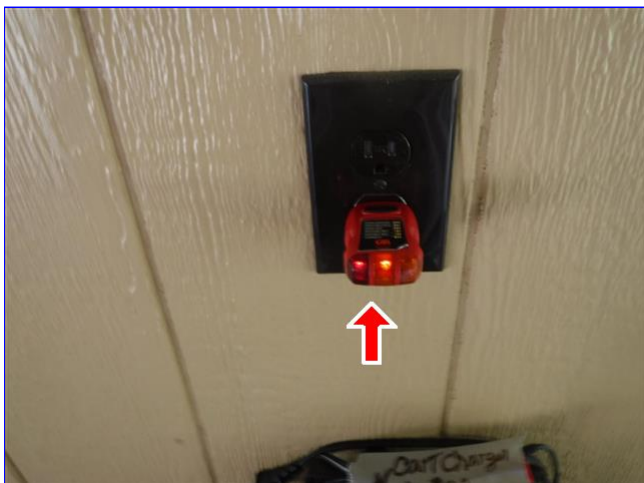
B. Item 8(Picture) Reverse polarity (garage)
