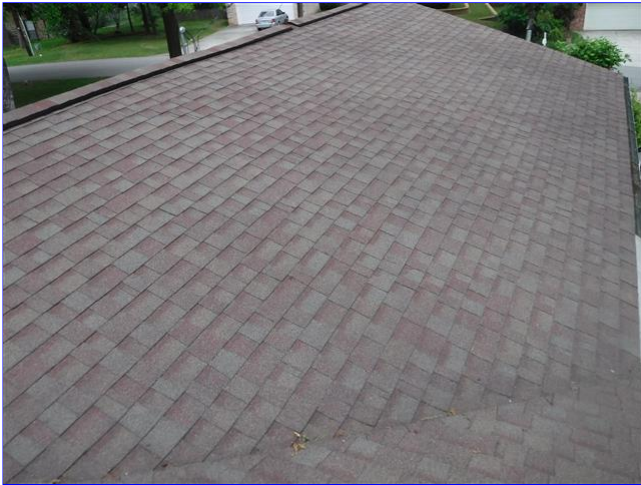
C. Item 2(Picture) View of roof.
