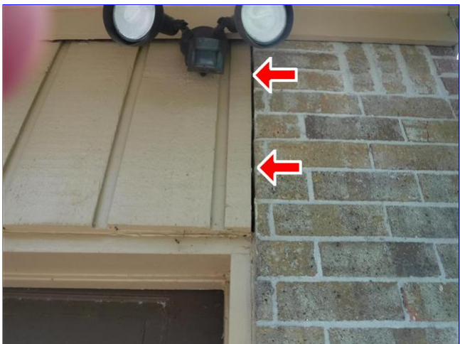
E. Item 3(Picture) This area needs to be sealed to prevent moisture and insect intrusion
