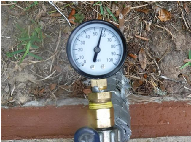
A. Item 1(Picture) View of measured water pressure
