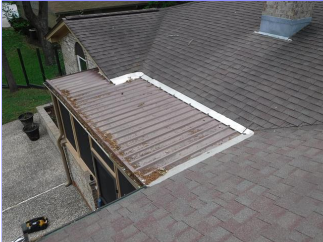
C. Item 3(Picture) View of roof.
