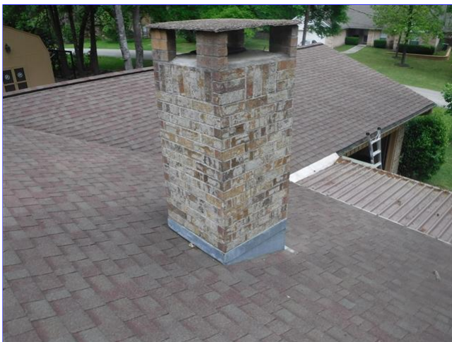
J. Item 2(Picture) View of fireplace chimney
