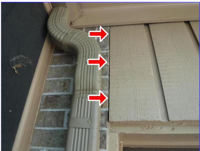
E. Item 4(Picture) This area needs to be sealed to prevent moisture and insect intrusion
