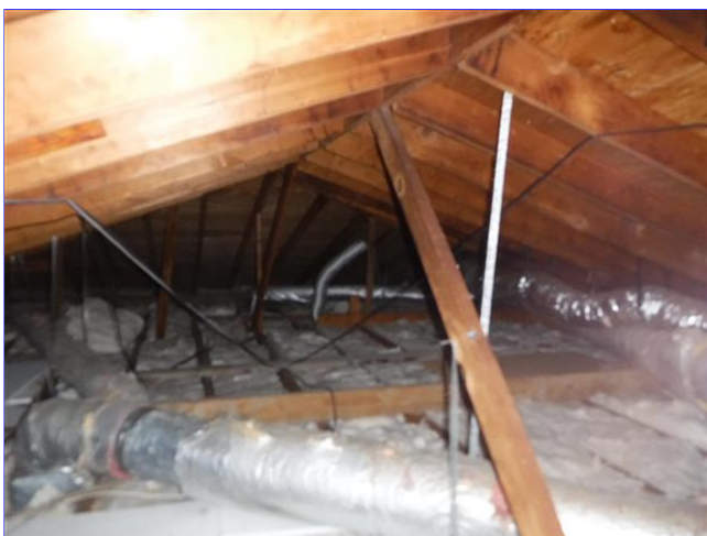
D. Item 2(Picture) Roof structure view.
