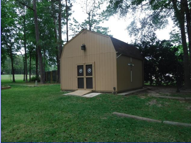
C. Item 1(Picture) View of outbuilding
