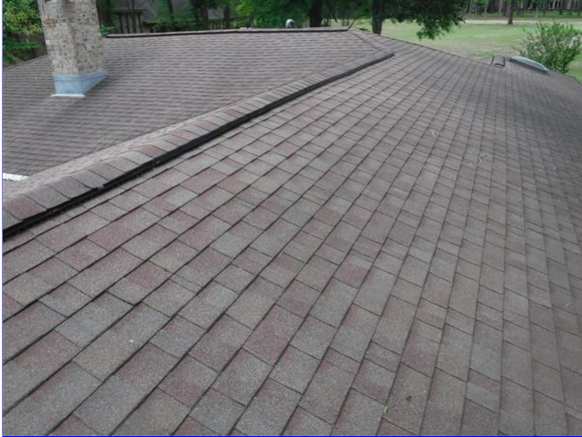
C. Item 1(Picture) View of roof.
