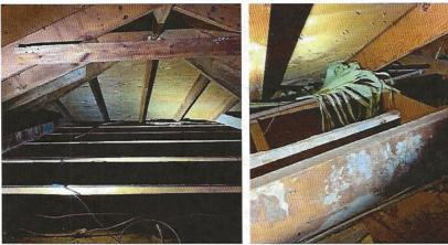
1. Insulation was observed to be of inadequate depth in the attic space (see photo). Typically insulation in the attic space should be even with, if not above, joists. Suggest adding insulation in attic space.
