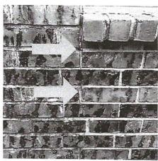
5. Separation was observed between the window frame and the brick wall on the left side of the home (see photo). Although this is indicative of foundation movement, excessive movement was not noted and the foundation appears to be operating as intended at the time of inspection. Recommend consulting with a qualified contractor regarding this condition.
