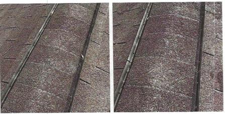
2. Damaged shingles were observed in one or more locations on the surface of the roof (see photos). Recommend consulting with a qualified roofer regarding this condition.
