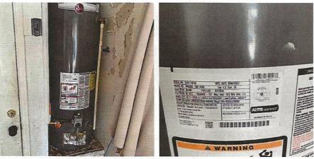
· 1. A drain pan is missing underneath the water heater (see photo). Recommend adding a safety pan.
